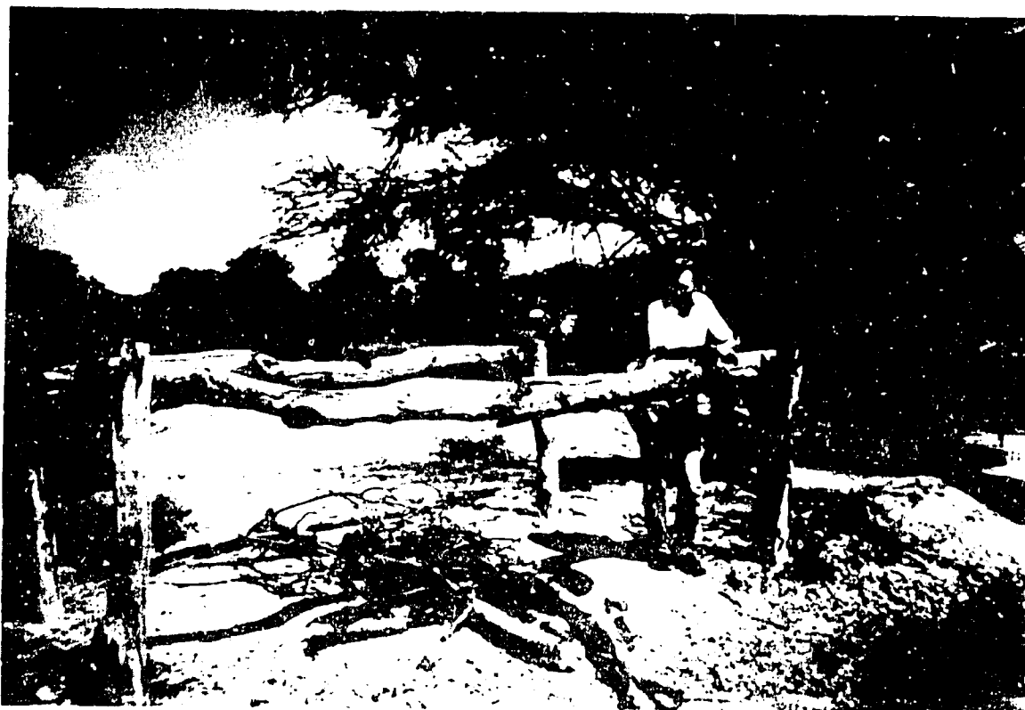
Photo 15. Hand-dug Well at Samecupi Abandoned as Bedrock Encountered without Finding Water
