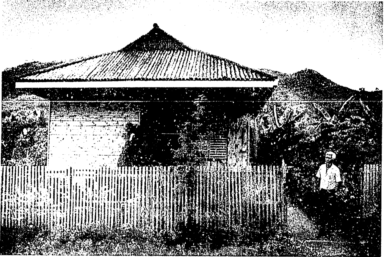
Top: A completed MEREC demonstration house, built entirely with local building materials and incorporating resource-efficiency design principles, in Tacloban, Philippines.
