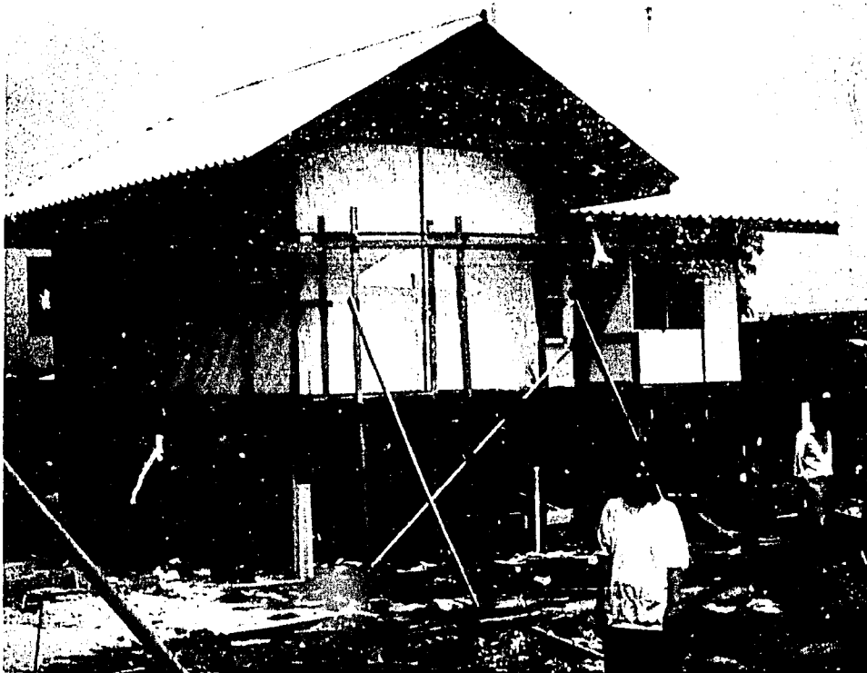
Above: A completed and occupied duplex MEREK demonstration house in Phuket. The demonstration houses incorporate local building materials and resource-efficiency design features, including biogas digesters, rainwater collection tanks, and natural cooling.
