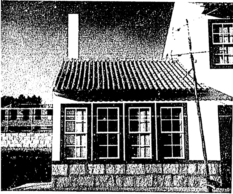
Above: A wing of a new school being constructed as part of a large educational complex for retarded children in Guarda. Guarda's MERECE design team introduced design alterations that led to incorporation of locally quarried granite and locally harvested wood into the building. The school also features wood window frames, wall insulation, insulated storm shutters, wood stove heating, and other MERECE principles.
