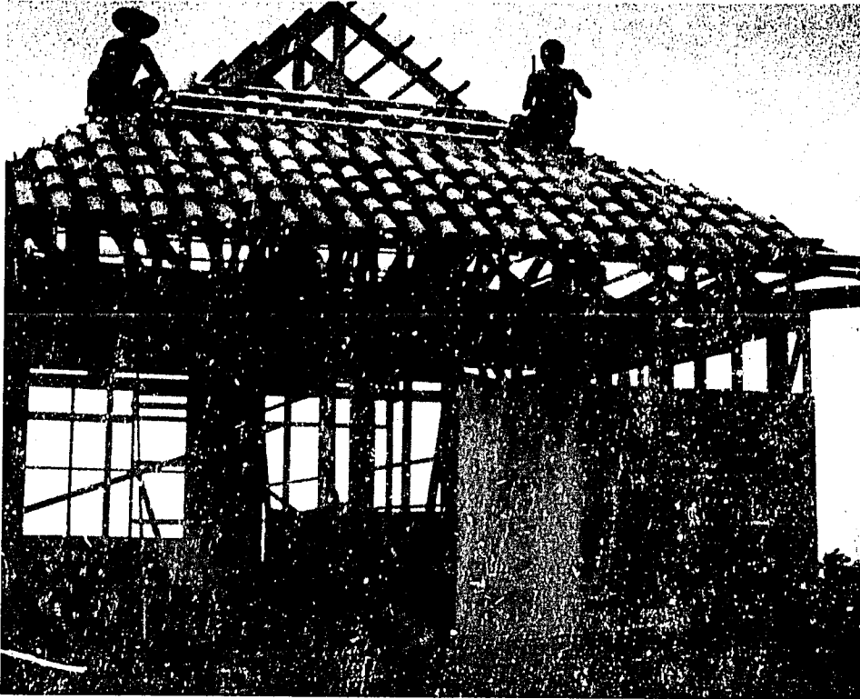
Under Tacloban's MEREC demonstration housing project, eight houses incorporating resource-efficiency principles and local building materials were designed and built. The upper photo shows one of the MEREC demonstration housing units under construction. The lower photo shows the counterpart conventional home of a family living near the MEREC demonstration houses. Upper photo by Tennessee Valley Authority.
