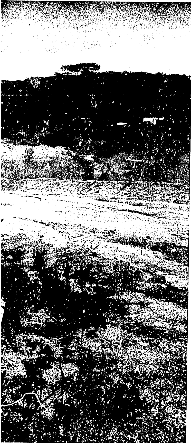
Left: A scene in an abandoned tin mine area being reclaimed under Phuket's MERECE demonstration as an urban resource for a variety of uses. Seen here are a drainage culvert and a road through the area that is under construction. The area to the right will be public parkland and will include a fishing pond.
