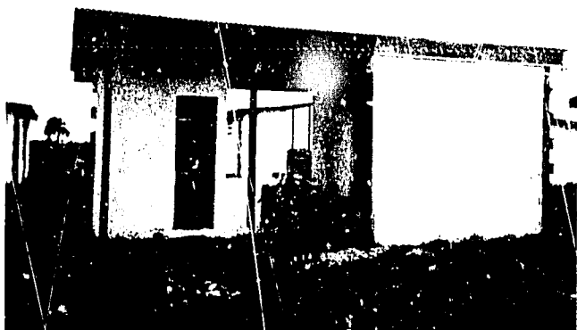
Figure 4. A core unit in the New Georgia sites and services project.
