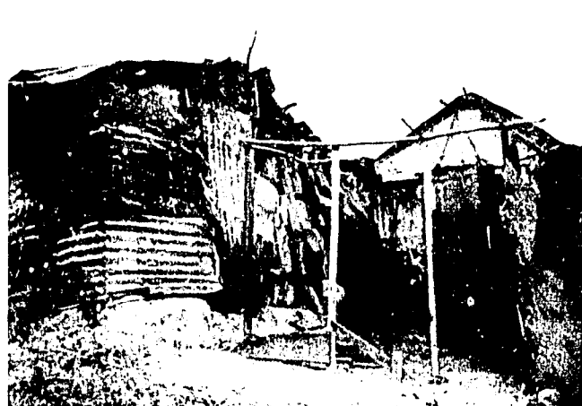
Figure 3. Housing of "below-average" quality in St. Martin.
