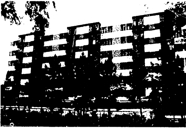
Figure 4. This is one of the better apartment buildings in urban China, in Harbin. These new units usually have two bedrooms, private kitchen, and western-style bathroom.
