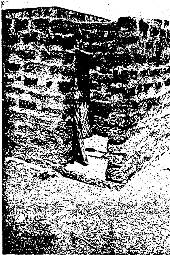
Photo 10. Latrine built with laterite blocks.
