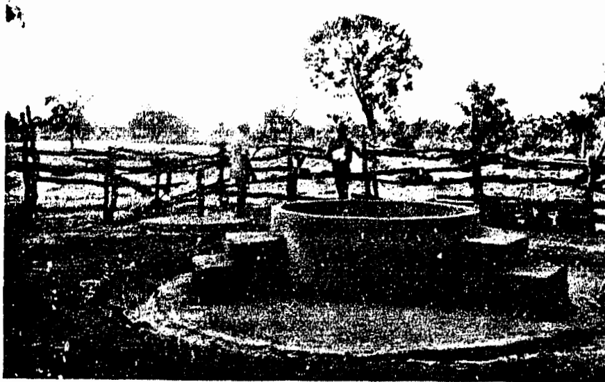
Photo 6. Large-diameter well with drainage system and fence. Pump has been removed.
