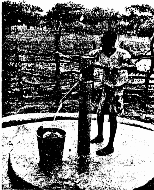
Photo 7. Project well with proper drainage system and fence.
