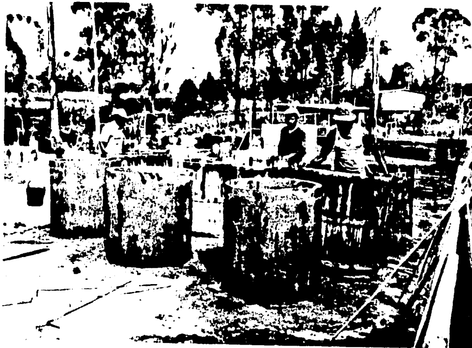
Photo 7. Production of well liners.
