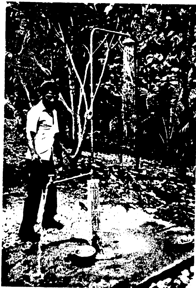
27. Public tap and shower installation.
