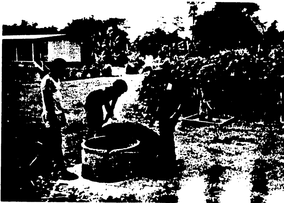
Photo 8. Dug well and offset handpump.
