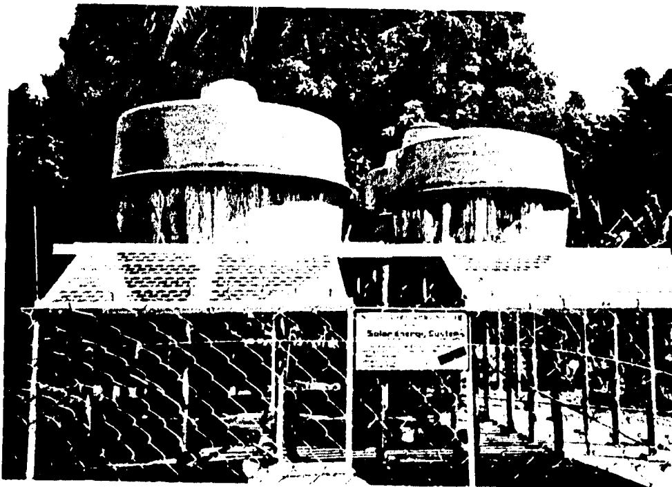
Photo 5. Fiberglass tanks and photo-voltaic panels.
