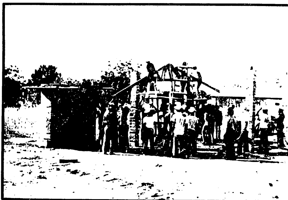
Photo 2. Trainees hoist the roof beam atop reinforced pillars to build the catchments hangar.
