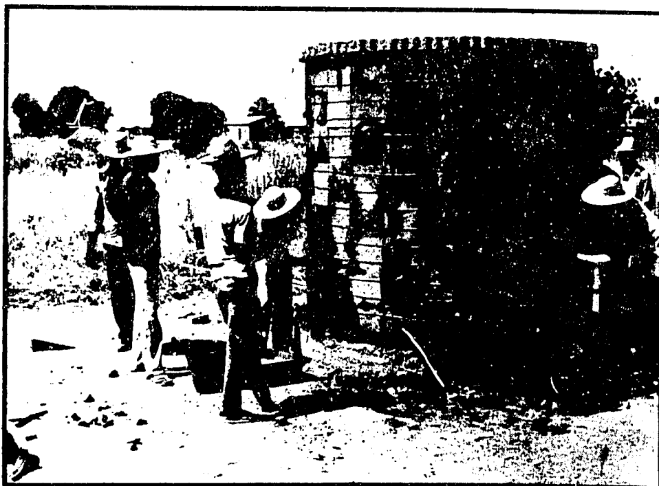
Photo 8. Trainees beginning to apply the exterior layer of mortar to the cistern.
