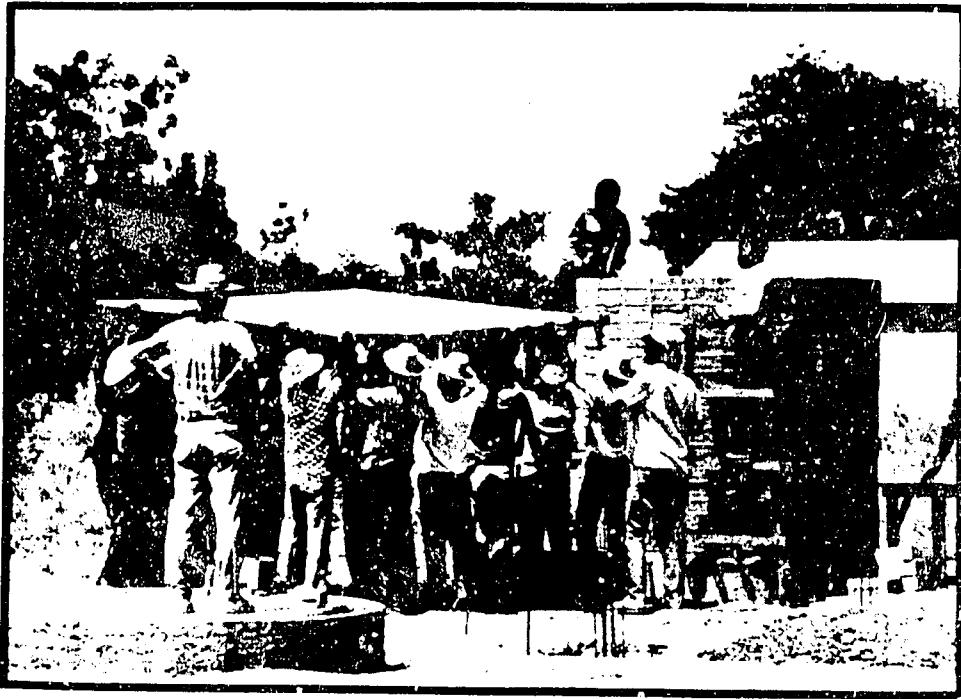
Photo 5. Trainees hoist the formwork to pour the cistern's cover slab in place.
