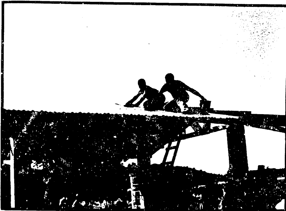
Photo 4. Trainees nailing the roofing on the water catchment hangar.
