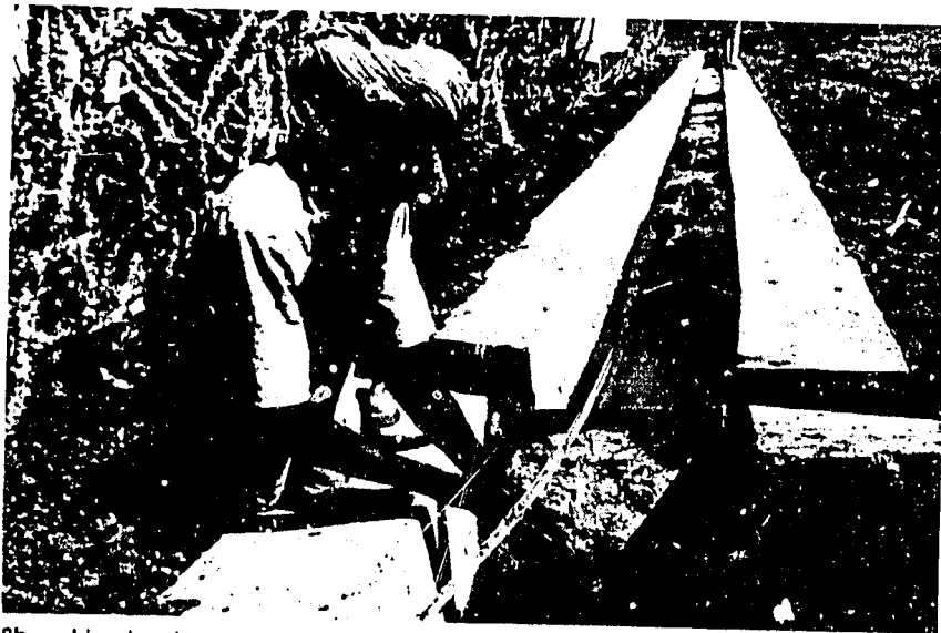
8b. Lined watercourse with stone slab check and earth plug in field outlet.
