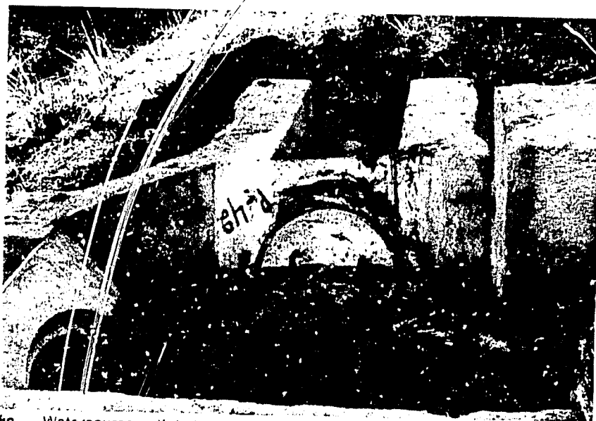
8c. Watercourse outlet structure with circular closure blocking outlet and allowing water to flow by.
