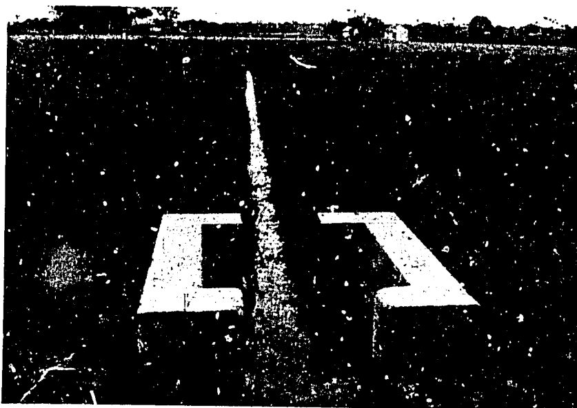
7b. Un-needed massive structure at end of lined channel.
