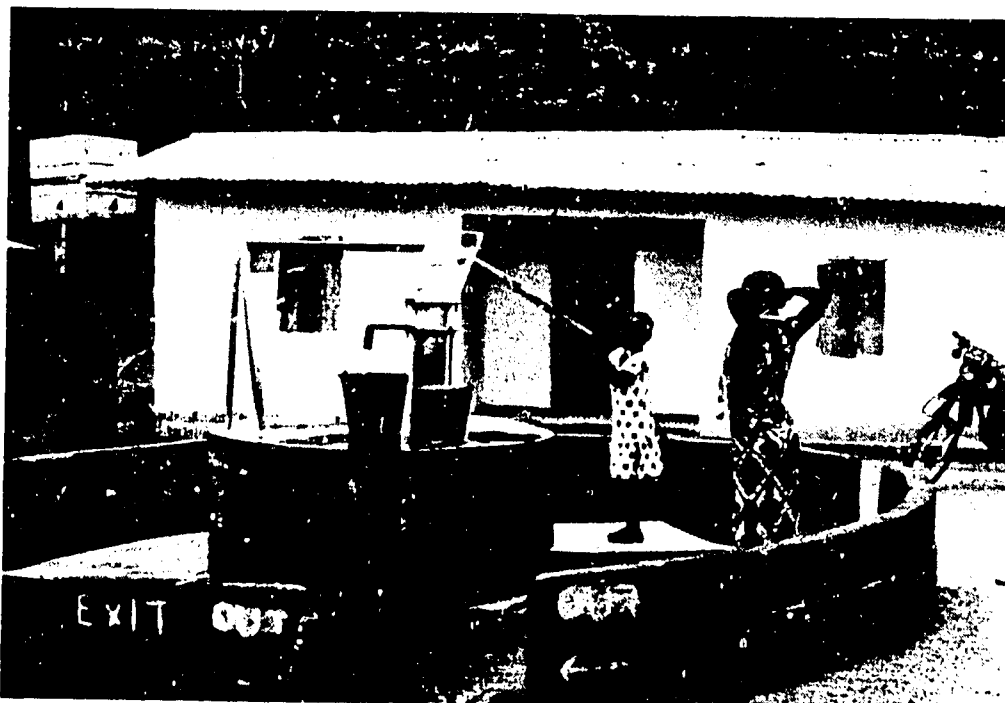
Photo 10. Well site with Mark IV handpump showing apron, pad for children to stand on, steel frame for mounting pulley, and concrete brick outer wall and surface drainage diversion.
