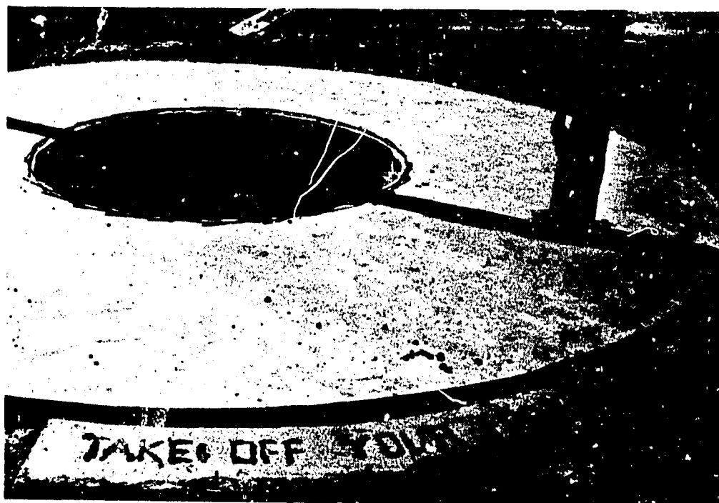
Photo 6. The poured-concrete apron with headwall and cover yet to be added.
