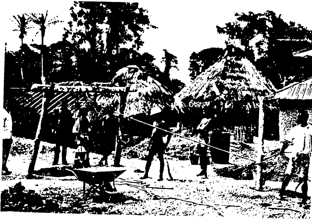
Photo 7. Well technicians and community members excavating well (note man in hard hat being lowered into the well).
