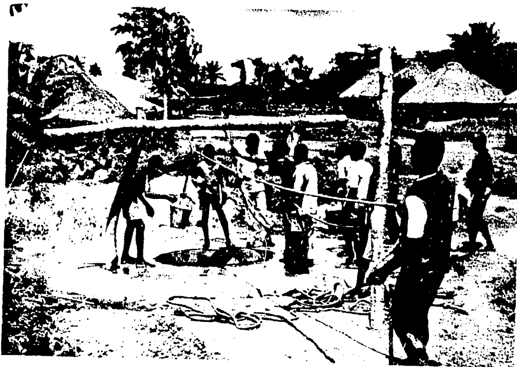
Photo 8. Well technicians and community members removing water from cassion to allow for excavation and cassion lowering.
