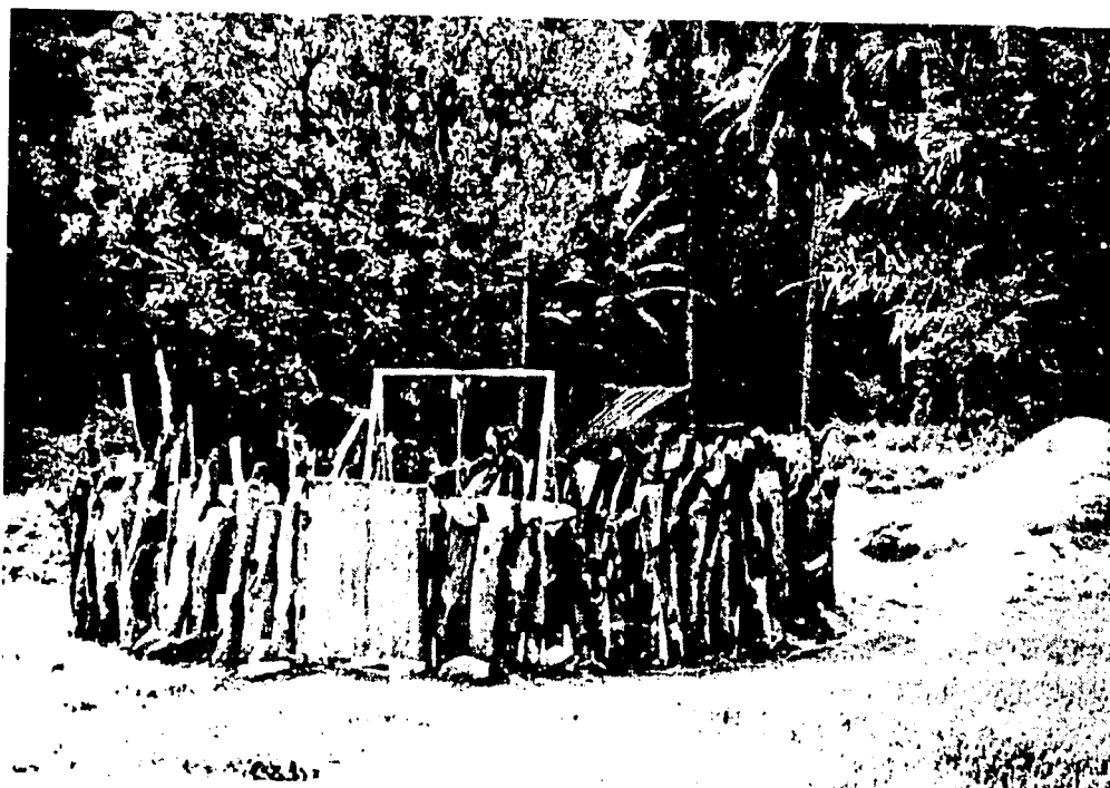
Photos 1-3. The MEP/CARE hand-dug wells feature locally designed and constructed structures and fences built from bamboo, bush poles, and timbers.
