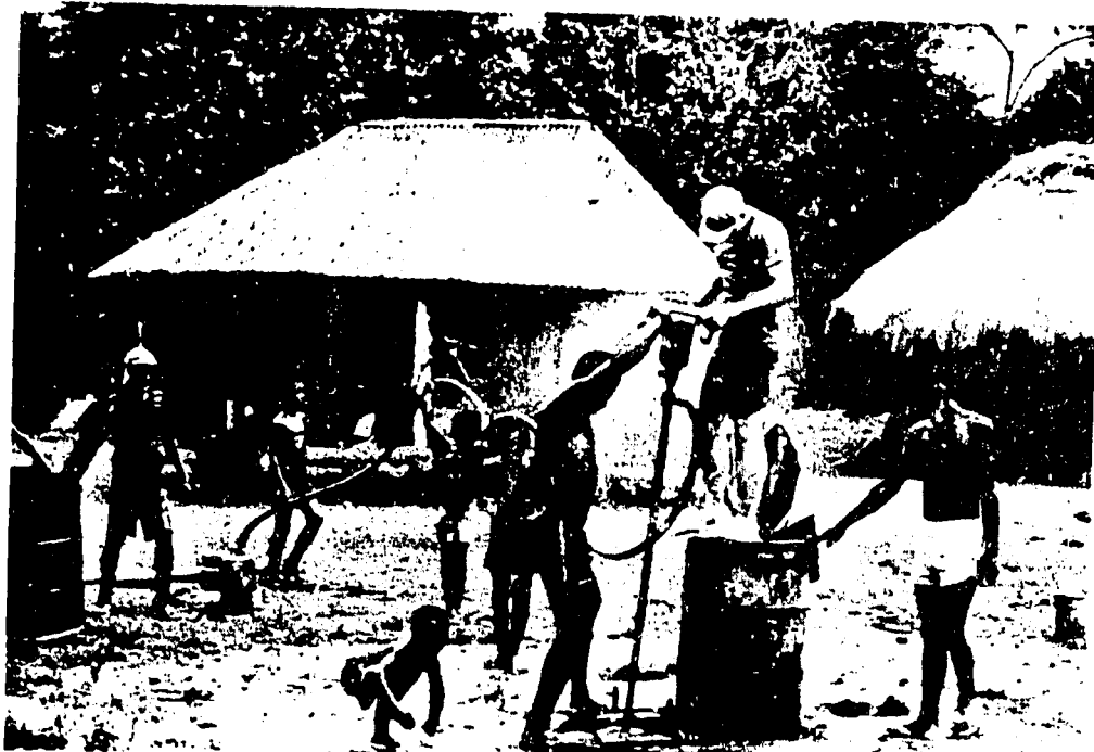
Photo 12. Well technicians test drilling with a hydro drill (water source in 50 gallon bucket, gasoline driven pump, and hydro drill).
