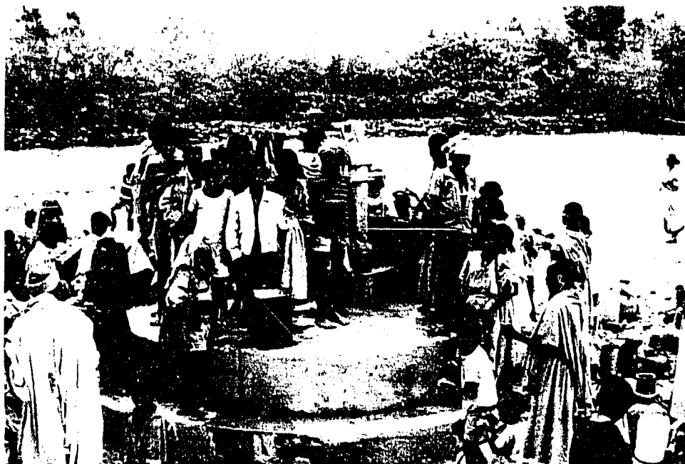
Photo 5. Handpump on a shallow well near Adwa camp. Supplied by UNICEF, this handpump provides the only source of water in the camp. The ICRC supplements the handpump supply with approximately 10,000 liters per day brought by tanker truck from Adwa town.
