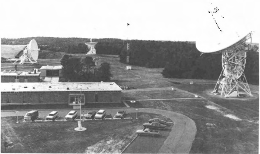
FIGURE 6-1 Satellite-receiving facilities are very expensive to build, but developing countries are now able to obtain satellite sensing data through both international data transfer arrangements and the development of multi-country regional receiving centers. (National Oceanic and Atmospheric Administration)
