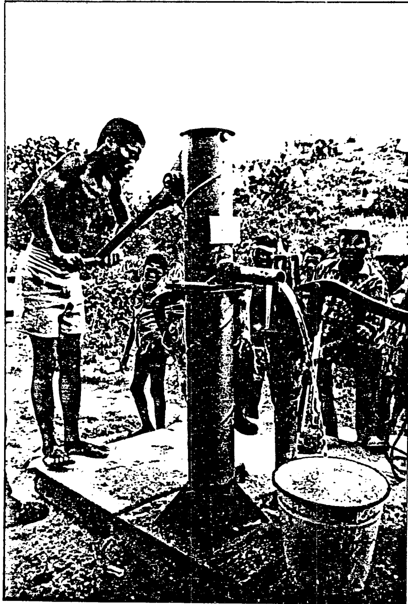
MALAWI HANDPUMP INSTALLATION AT TAIWAN
