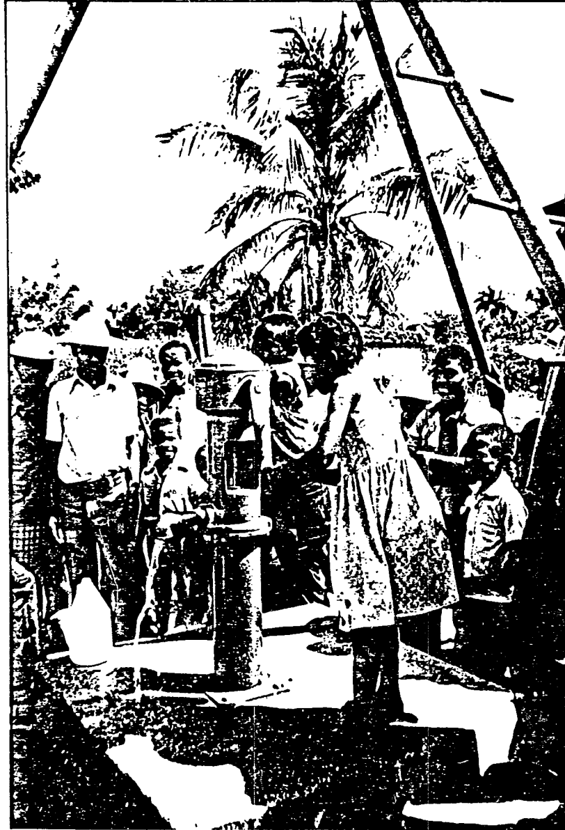
MONO HANDPUMP INSTALLATION AT MIZINE
