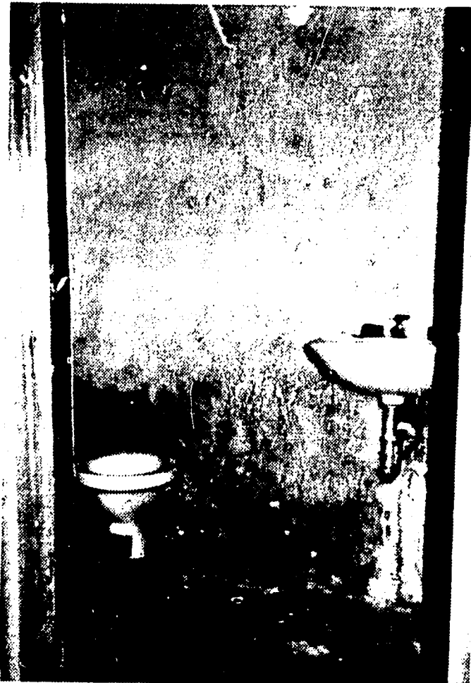
Imported ceramic fixtures installed in a shower/ bathroom combination
