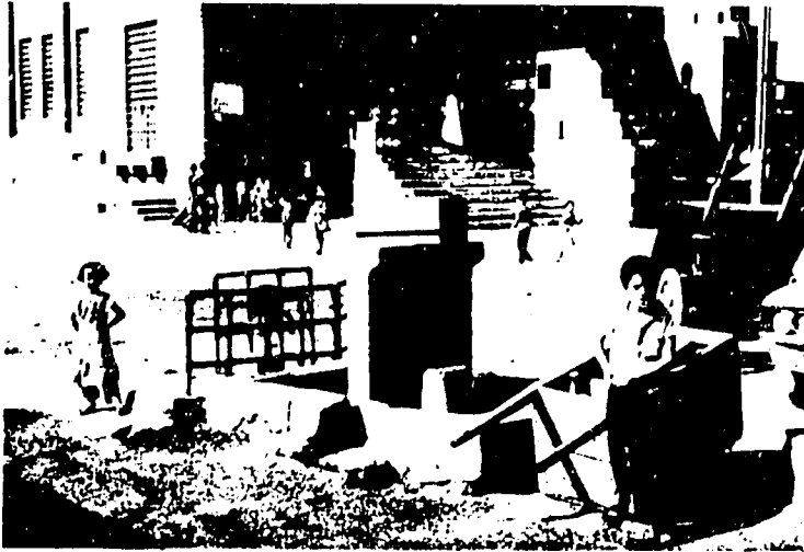
Inoperative Public Standpost
