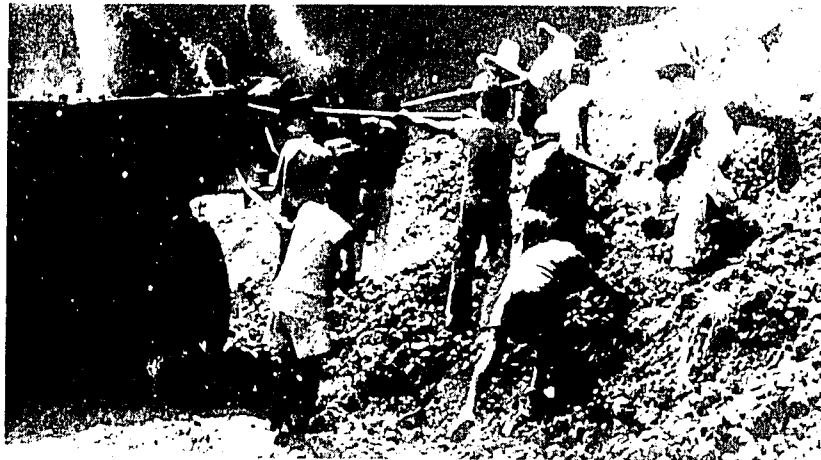
Figure 4. One of the main features of appropriate technology is labor-intensive practices, such as shown here.
