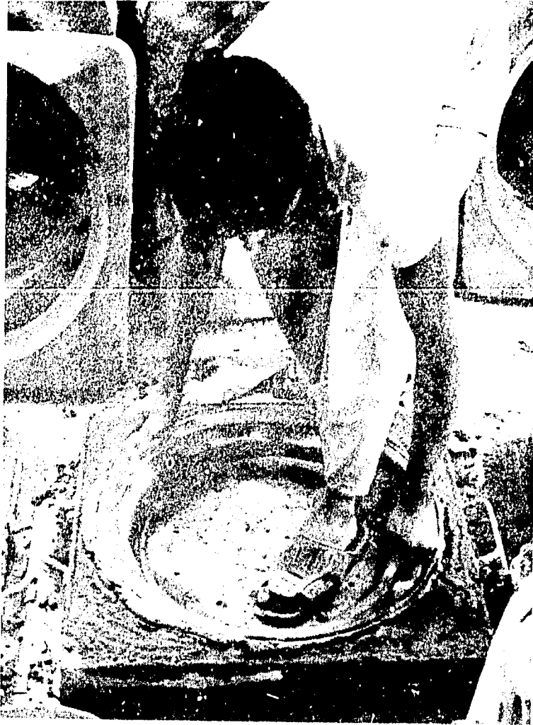
Figure 3.13. Placing the panel ring form in the panel to shape the mortar. Notice the handles on the ring.
