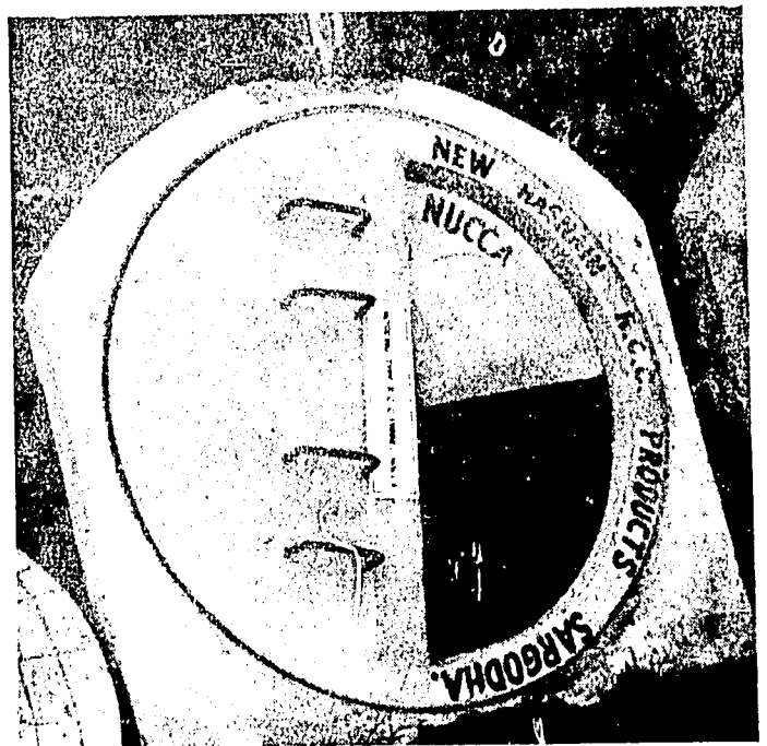
Figure 5.7. Large circular rotating turnout with half-circle cutout.
