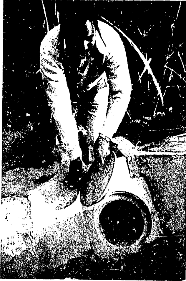
Figure 4.2. Turnout panel installed in a lined channel.
