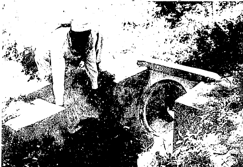
Figure 4.3. Circular concrete check and turnout installed with brick masonry in an earthen channel.
