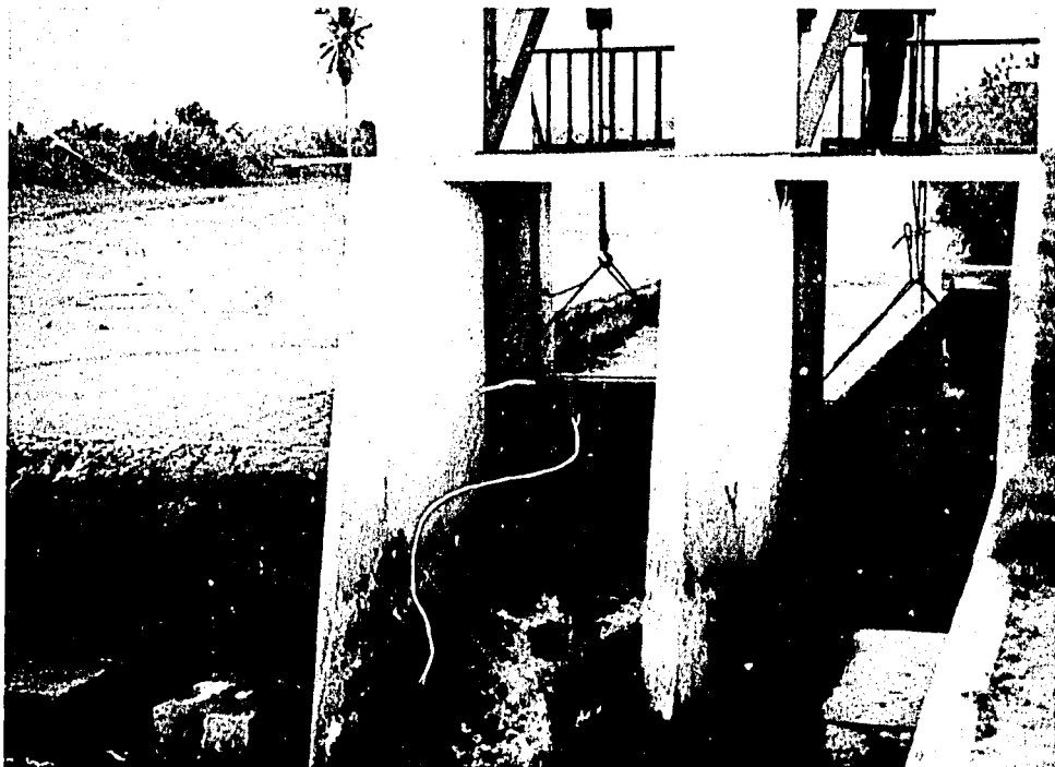
Photograph 30. - Looking upstream from below the sluice gates at Banga River Diversion Dam during a sluicing operation.
