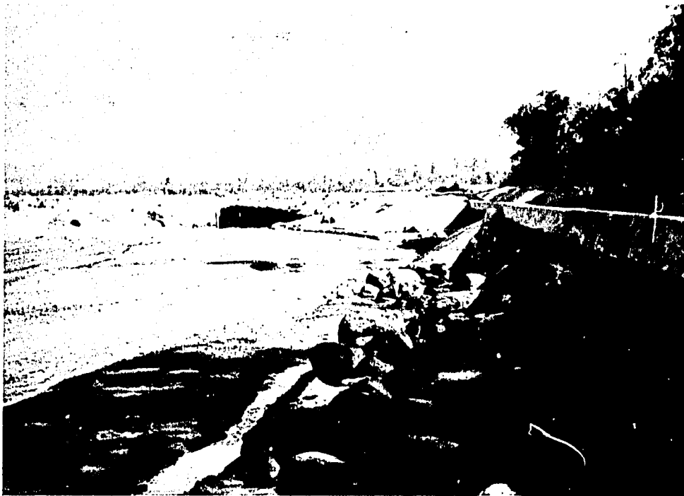
Photograph 8. - Upstream view from near headworks at Santo Tomas River Diversion damsite showing type of rock used for riprap along diversion wall.
