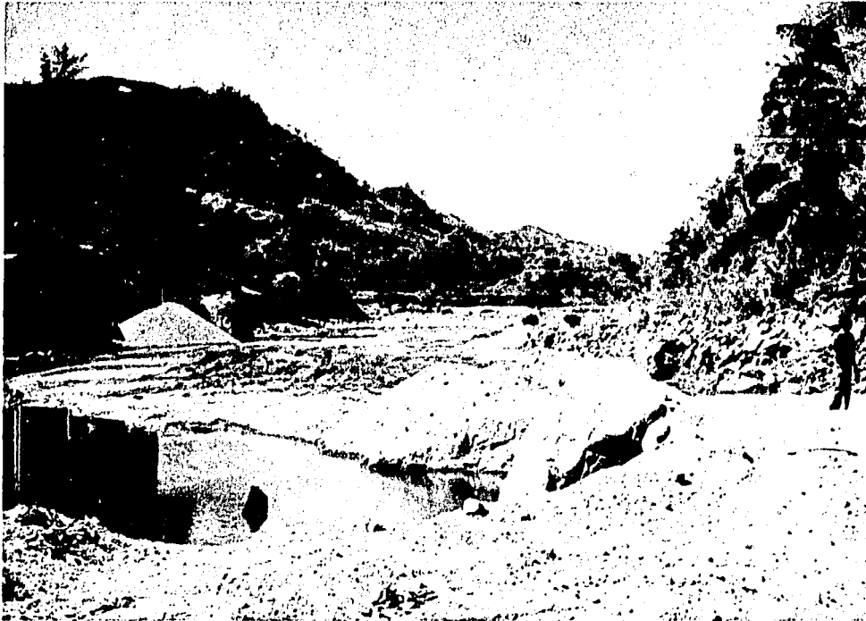
Photograph 9. - Looking downstream on Santo Tomas River from above sheet piling used the past year for diversion.
