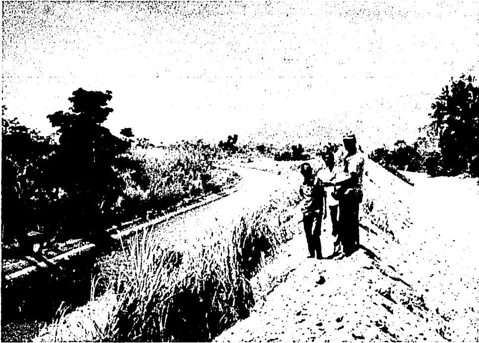
Photograph 17. - Canal below Santo Tomas River Diversion showing type of material cleaned from concrete-lined canal section.
