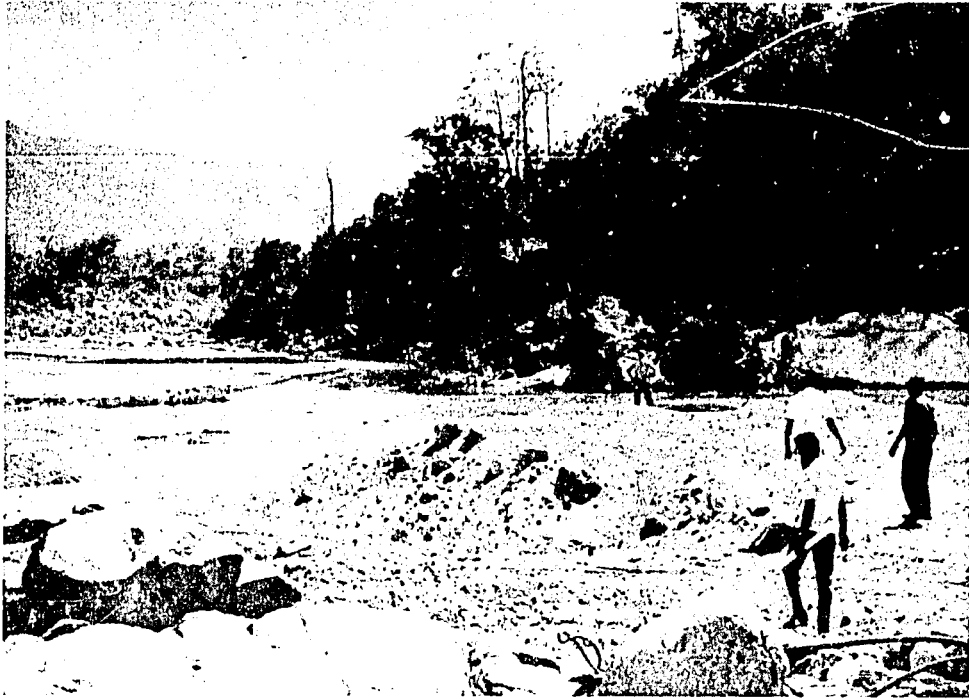
Photograph 15. - Looking across Santo Tomas River from right bank showing left bank abutment to a proposed diversion dam-site about 180 meters above the old diversion dam-site.
