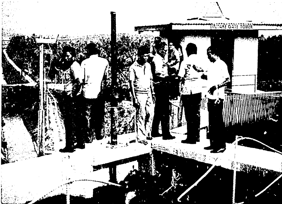
Photograph 25. - Intake to powerplant below Marbel River Diversion Dam.
