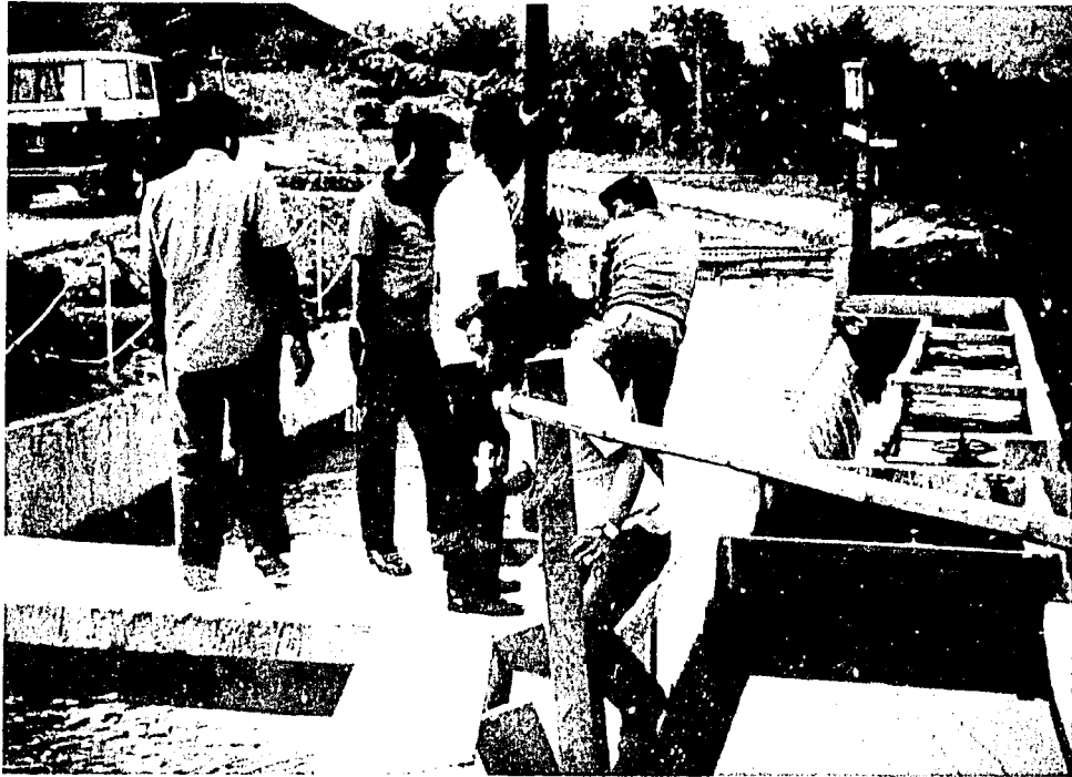
Photograph 24. - Looking up the canal several miles below Marbel River Diversion Dam at the powerplant intake structure showing the water being skimmed used for cooling
