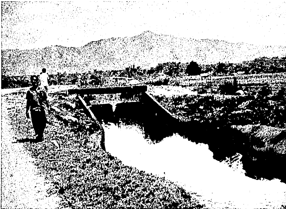
Photograph 18. Drop structure on canal below Santo Tomas River Diversion damsite.
