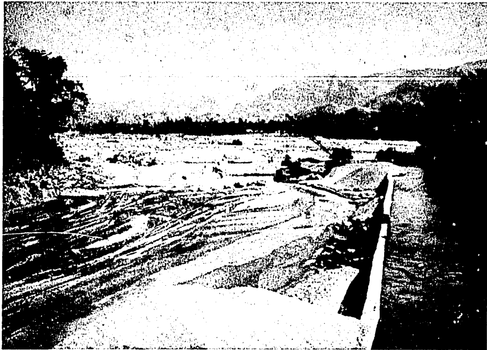
Photograph 7. - Upstream view from near headworks at Santo Tomas River Diversion damsite showing removal of sheet piling.
