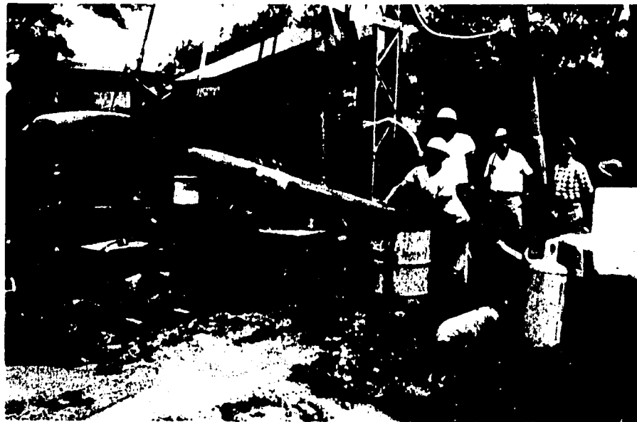
11. Well drilling at Site 13 (Galo). Costs of well drilling, development, and pumps were borne by farm owners.
