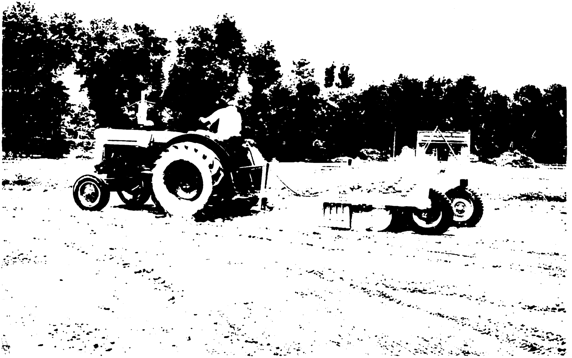
Machinery such as this tractor and scraper are important ingredients to a successful land leveling construction project.
