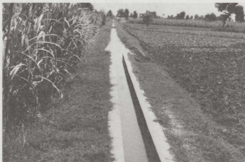
Lined and unlined sections of an improved watercourse.
