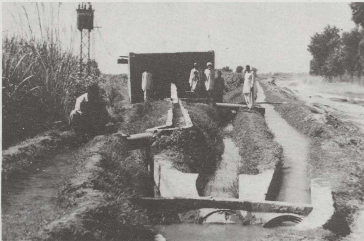
A tubewell supplies additional water to a farmer's private ditch (left) adjacent to an improved watercourse.
