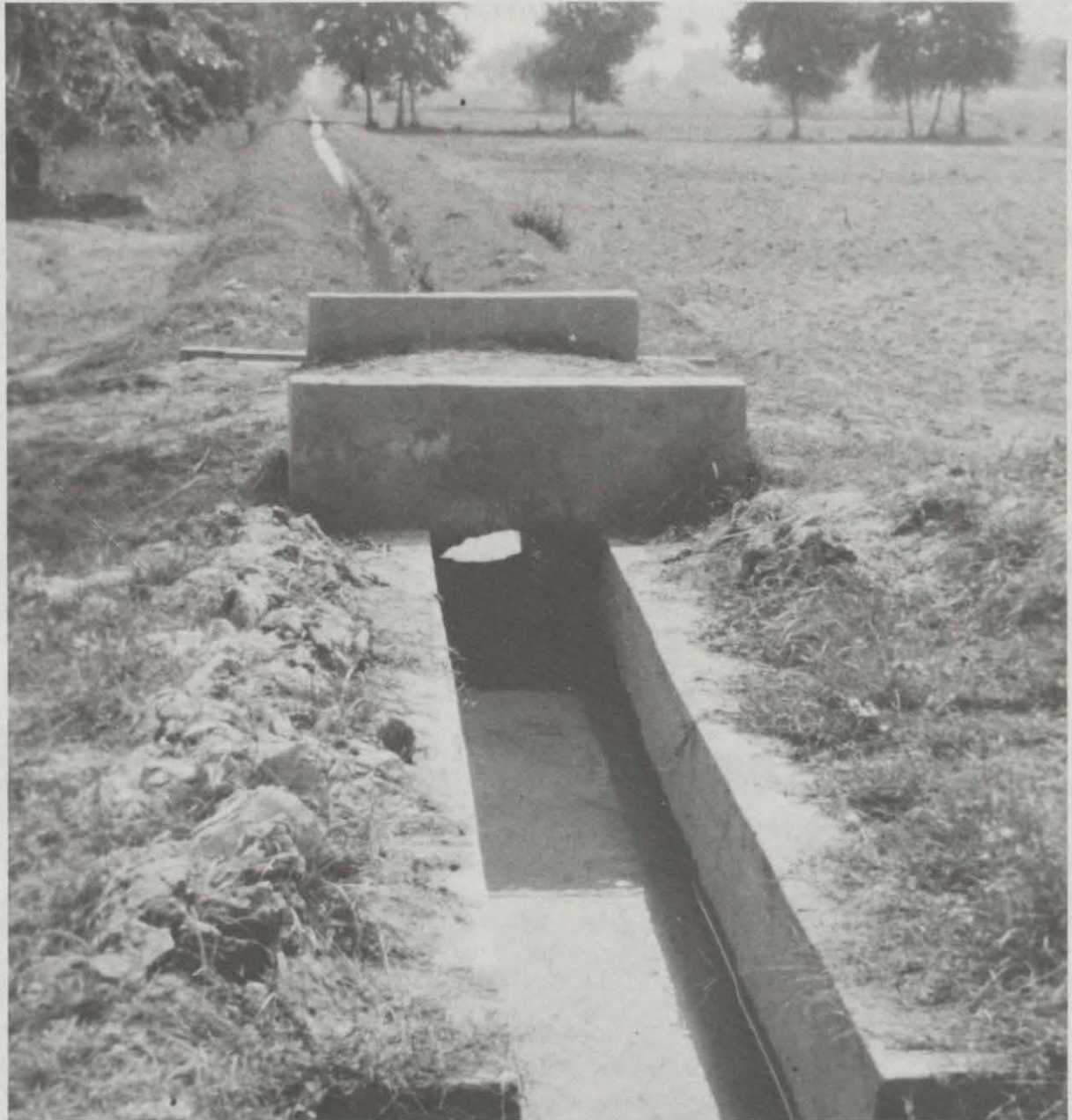
Concrete culvert crosses an improved watercourse.
