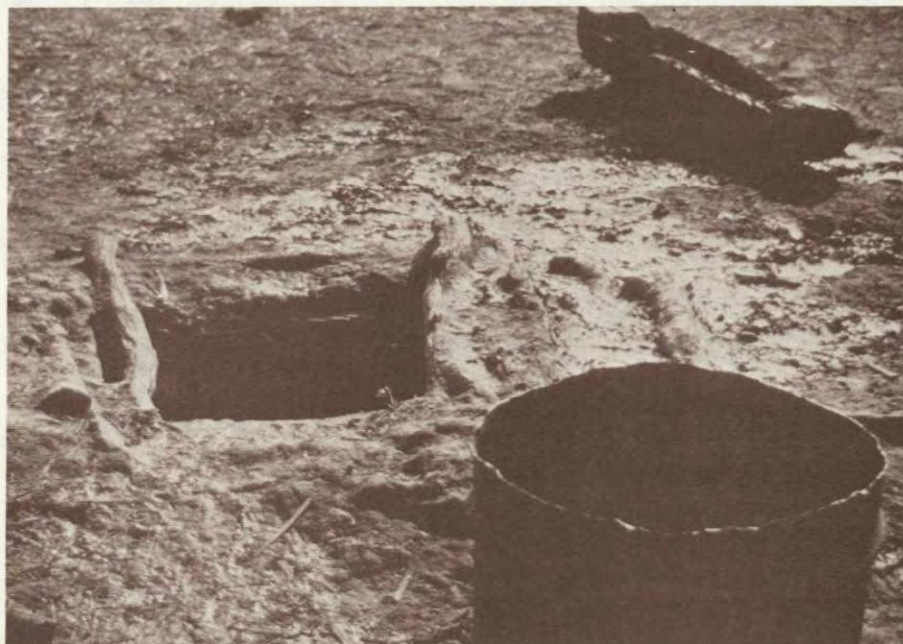
Improperly placed and constructed wells in the Senegal River Basin lead to contaminated potable water supplies. Note animal trough in the background.
