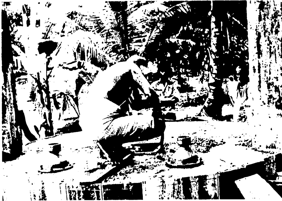
FIGURE 19. FINAL TOUCHES ADDED TO THE SLAB AT SERUPITA (SRI LANKA)
