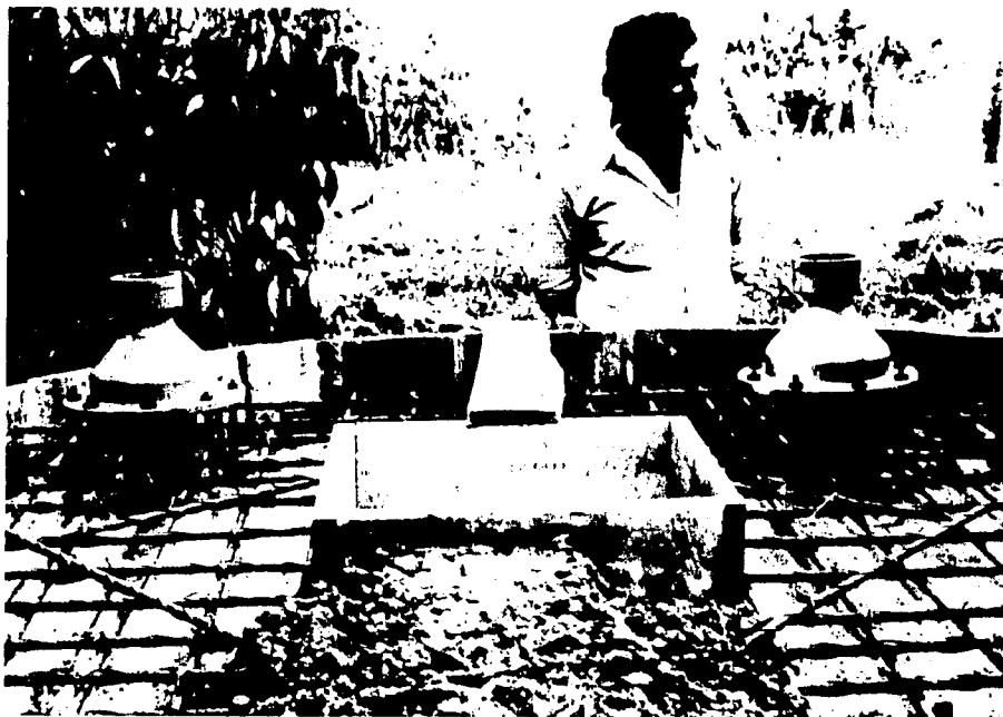
FIGURE 18. SLAB FOR AID HAND PUMPS (SRI LANKA)
