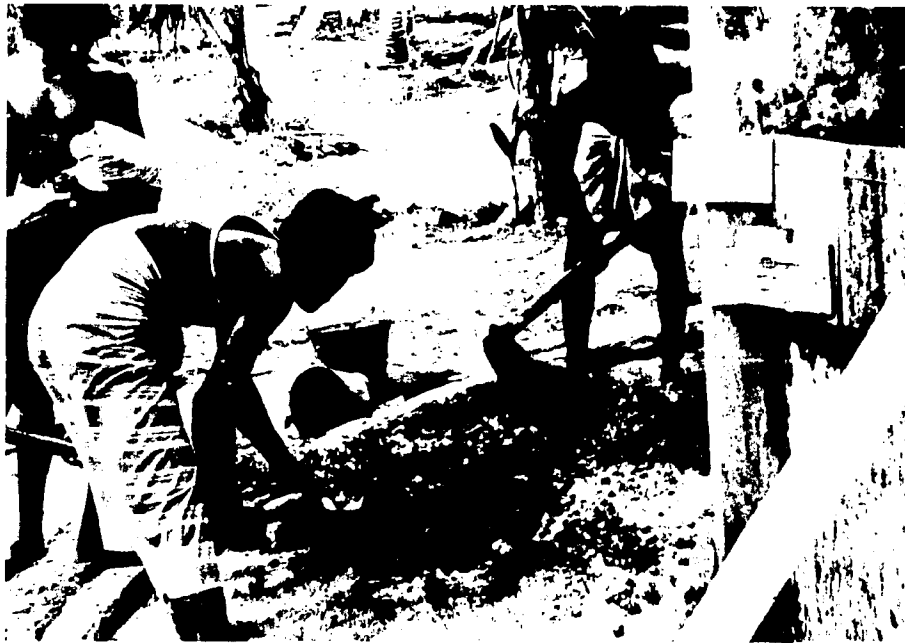
FIGURE 17. SERUPITA, SRI LANKA VILLAGERS HELP DEVELOP AN EXISTING WELL FOR INSTALLATION OF TWO AID HAND PUMPS
