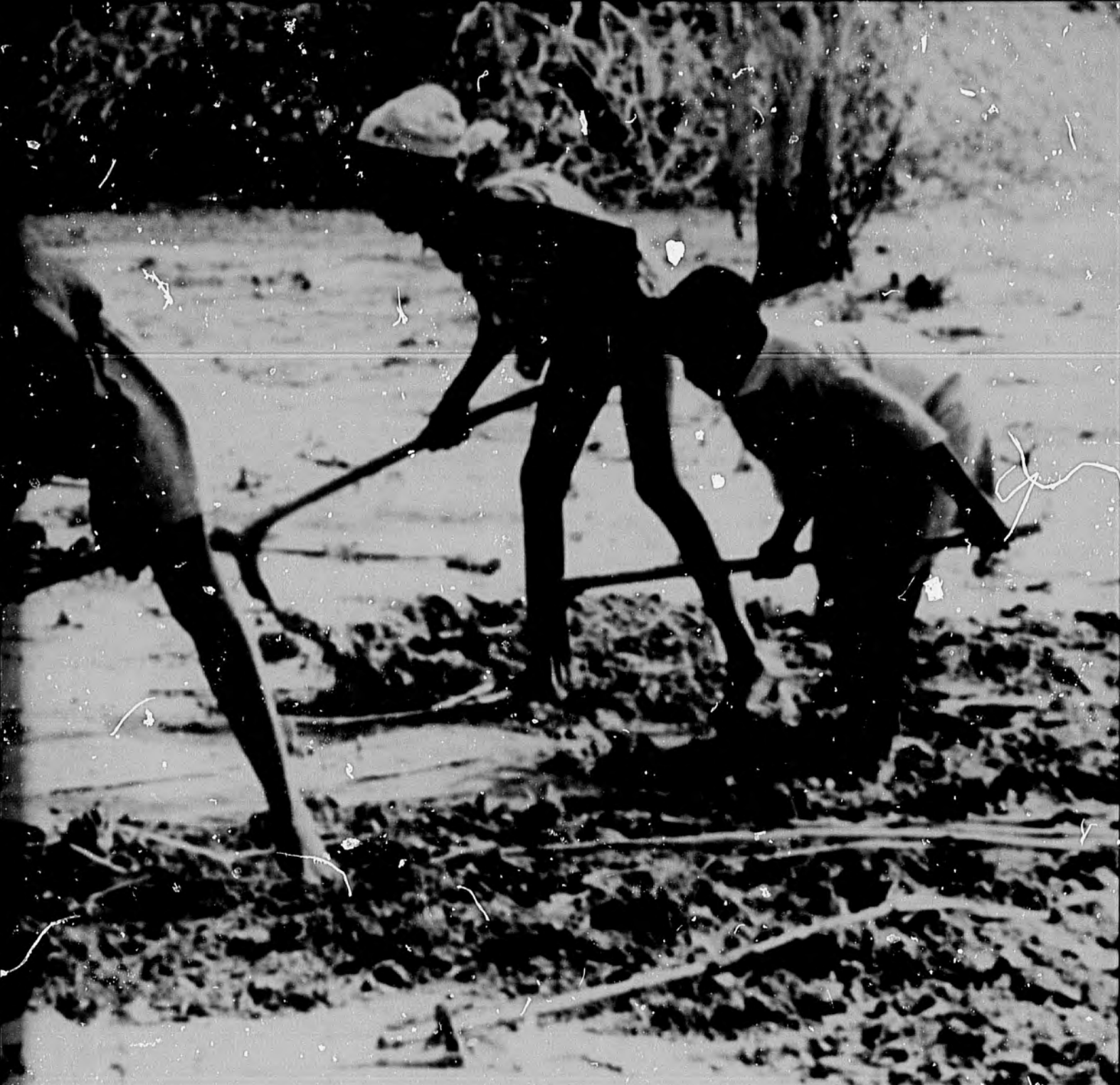
Where mechanized equipment is not available, a start at land leveling can be made with hand tools to clear away gross irregularities.
