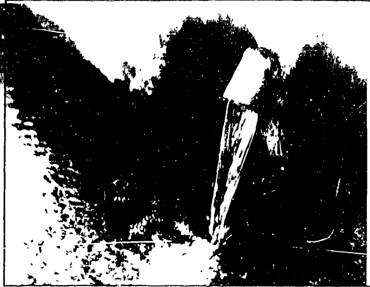
Springs were improved at 139 sites so that the water would flow through a pipe and into a concrete trough
