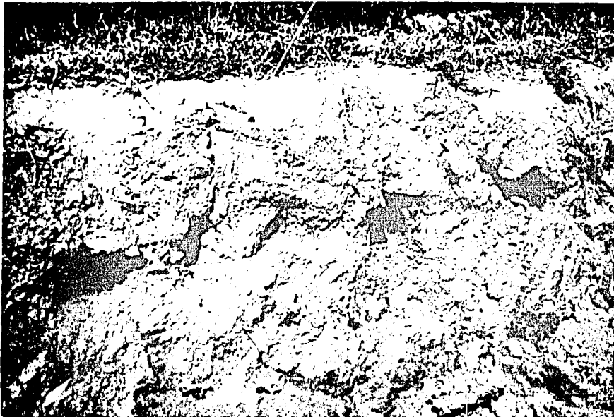
Figure 8. Rat burrows inside a watercourse bank exposed by excavating the inner portion of the bank.
