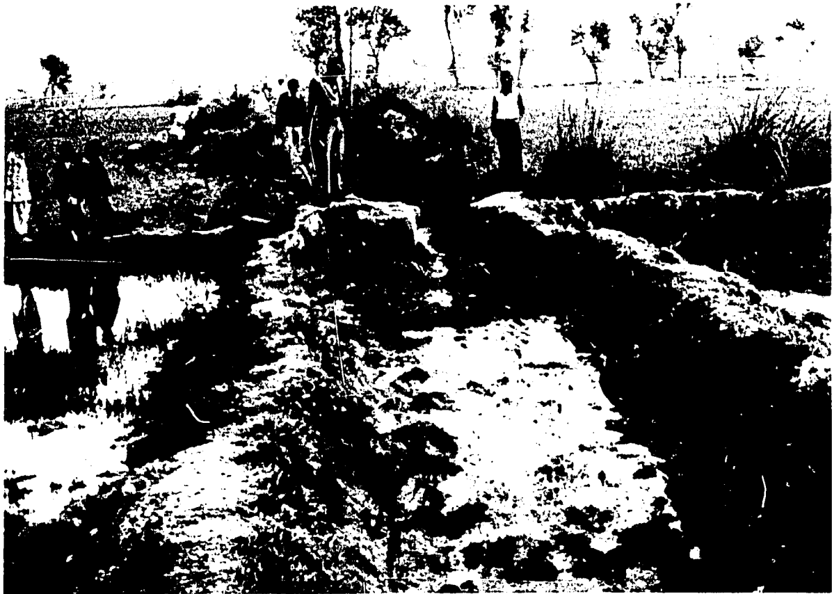
Here is a watercourse before it has been improved. Weeds and silt along with narrow banks have contributed to the overtopping, seepage and consequent loss of water.
