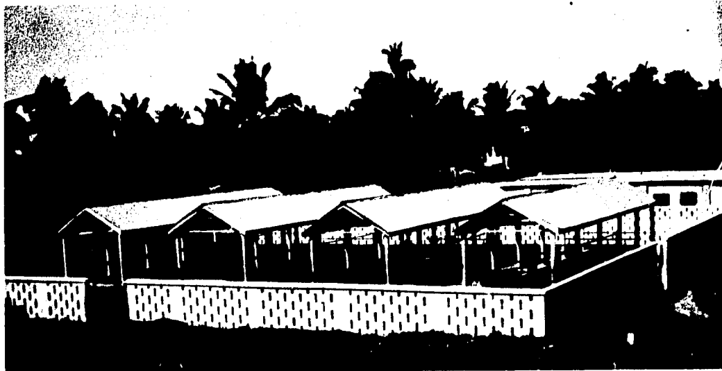
Figure 18. Today is not market day at this neat little arrangement in Anomabu. Note openness which allows free circulation of air - so important in the humid tropics.
