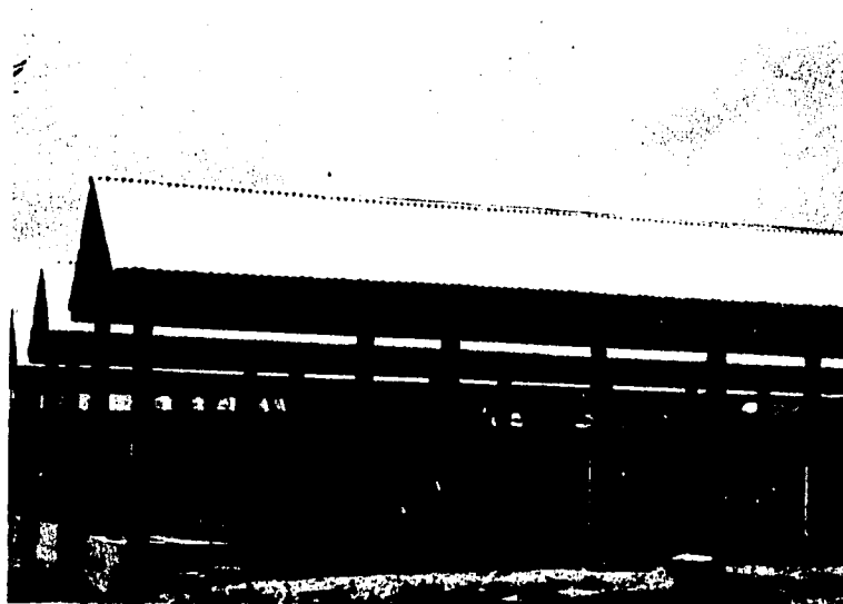
Figure 21. Here are newly constructed stalls at Kukurantumi. Stalls are divided with wooden rails and posts treated with creosote preservative.
