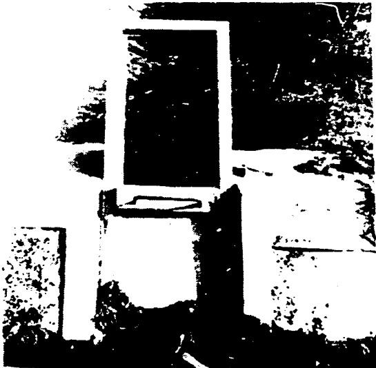
B. Inclined concrete sliding turnout (nakka) designed by Bill Hart for trapezoidal channels.
