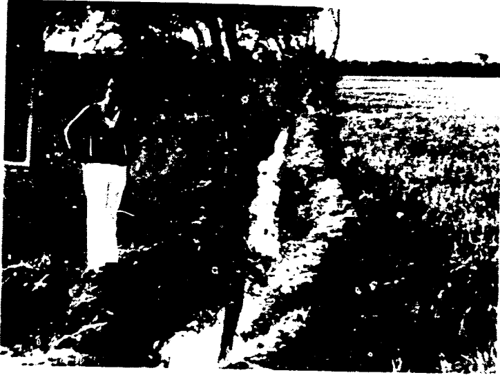
A. A typical branch watercourse showing grassy, porous banks. Note tree growth that consumptively uses water and occupies croppable areas (Mona Irrigation Project TW-78).
