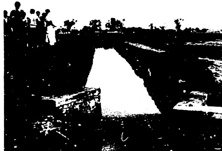
D. Settling basin to trap sand immediately downstream from Mogha shown in Photo C above.
