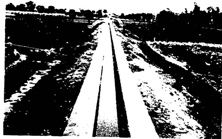
D. Rectangular brick masonry channel lining on Main 1 of tubewell 78 watercourse.
