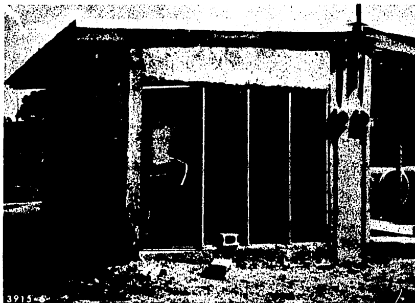
(b) Roughed in, steel-framed 200 square foot core
