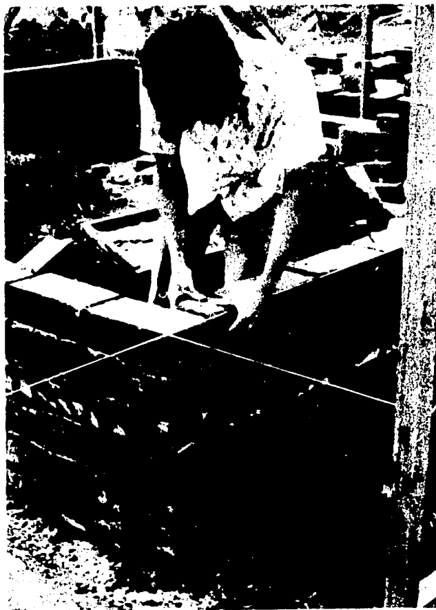
(a) Soil-cement (9/1 ratio) blocks being placed
