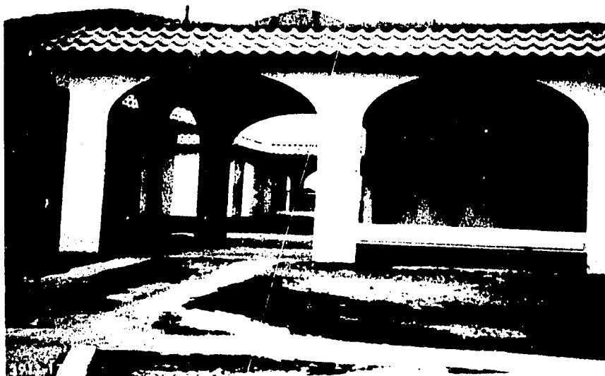
(b) Simulated tile roof of cast concrete
