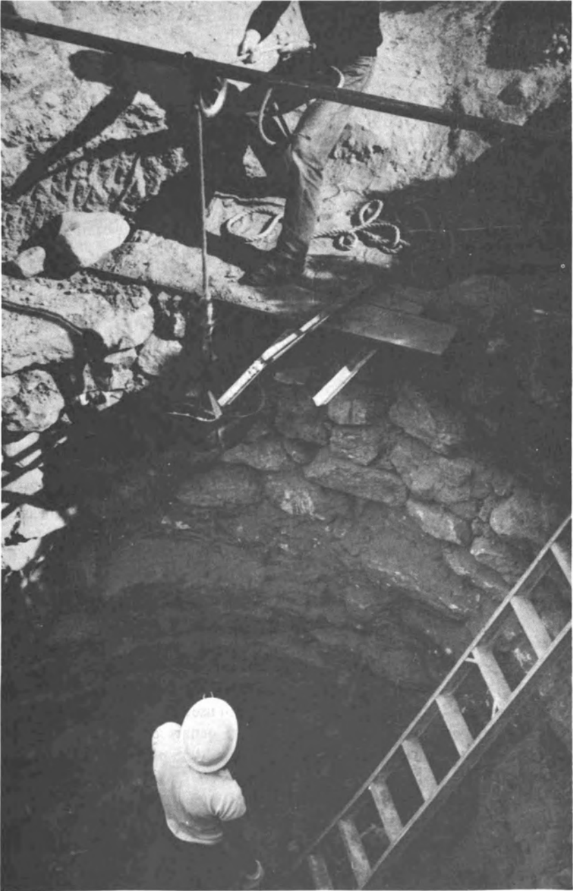
FIGURE 33 Excavation of a dug well in the Negev Desert. (U. Nessler)
