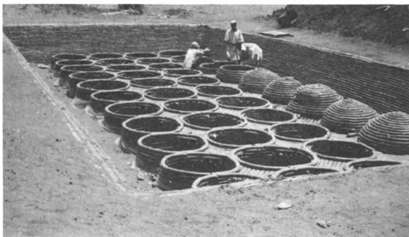
FIGURE 11 Capping 2-m-tall internal water-storage cells with soil-cement-filled sausages (FIGURE 12). The area will next be back-filled with sand. This technology requires only a spade, funnel, carving knife, and mallet. Kordofan Province, Sudan. (M. G. Ionides)
