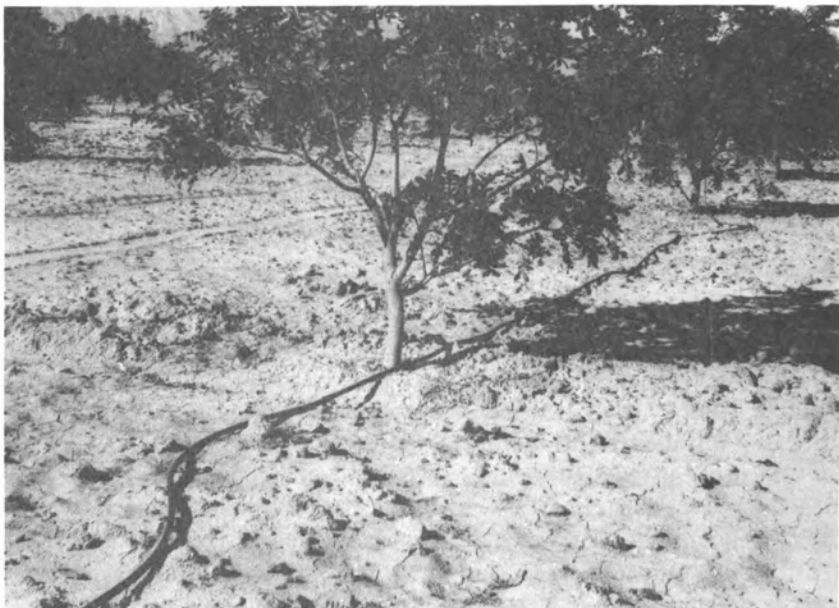
FIGURE 57 Trickle irrigation system in California, USA. Pipes lead the water to emitters beside the trees. (F. K. Aljibury)
