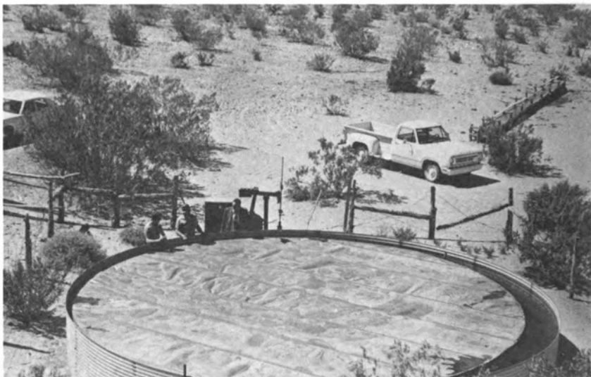
FIGURE 43 Floating foam-rubber sheet (9 m diameter, 5 mm thick) covers a water-storage tank near St. George, Utah, USA. Experience to date suggests that the cover will last 10 years with an evaporation-control efficiency of 80-90 percent. Estimated cost of the water saved in a 120-cm/year evaporation zone is US$1.80-$2.00. (U.S. Department of Agriculture)
