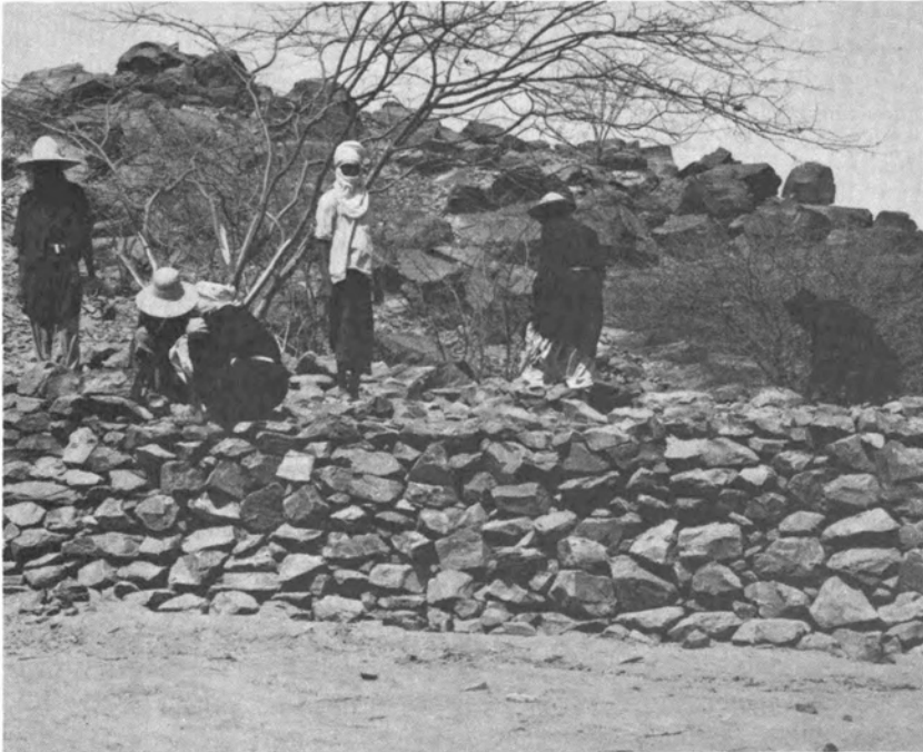
FIGURE 19 In 1972 near the small town of Tchirozerine (close to Agades), Niger, West Africa, Touareg nomads build a rock wall to capture flood waters. The soils here absorb little moisture, and the rainfall runs away in flash floods. Using stones gathered from the fields, Touareg workers built eight 1-m-high walls across the plains so that rain is retained, and absorbed by the soil. When summer showers fell in 1973, the water retained by stone dams and walls flooded nearly 1 square mile on the plain and grass flourished—extraordinary events in that area. (Oxfam-America)
