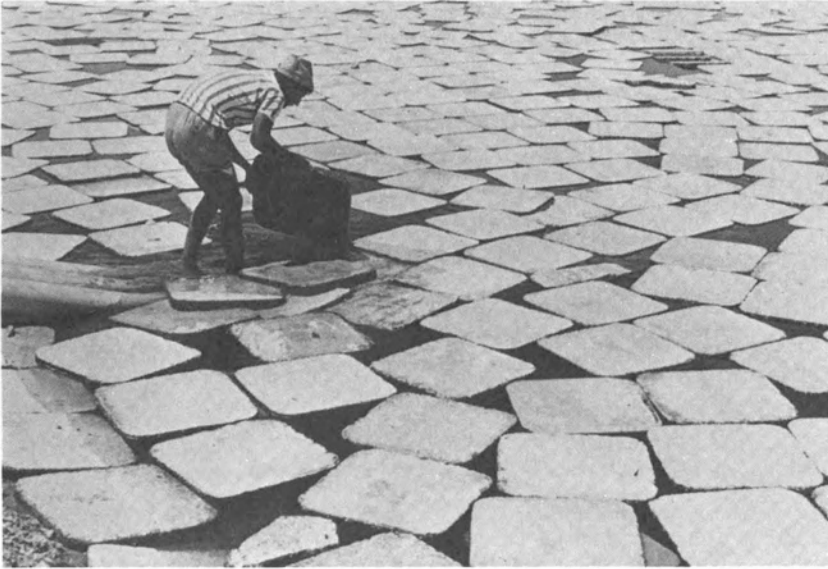
FIGURE 42 Protective covering of molded, lightweight, concrete slabs cut evaporation by an estimated 80 percent recently in full-scale tests on two reservoirs in Ovamboland, South-West Africa. Engineers cover reservoirs with 24-in 2 , 2-in thick floating slabs of polystyrene, sand, and concrete. Exposed surface of each slab is painted white to reflect the intense sun rays, which hasten evaporation.
