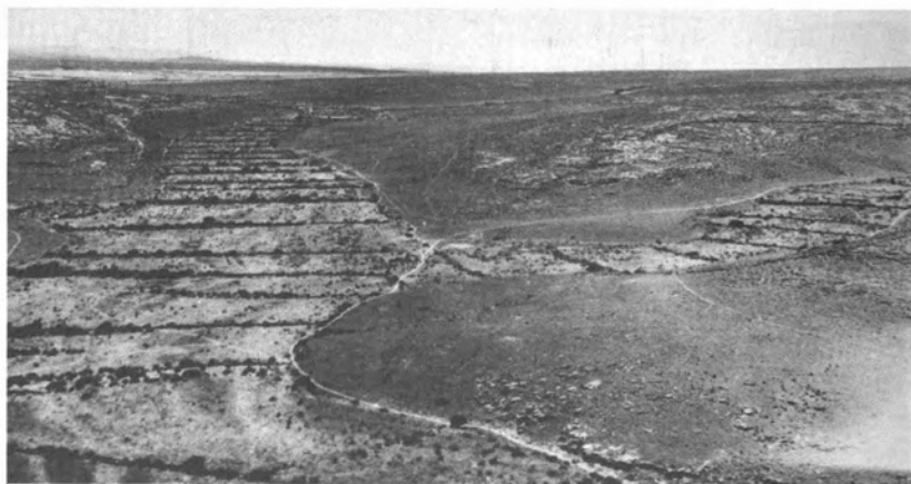
FIGURE 18 Man-made terraces (reinforced by unpalatable bushes) built in ancient times to slow down and capture floodwaters in this wadi in the Negev. Built thousands of years ago, some are still used for farming by Bedouins. Terrace walls are 10-50 m apart and about 30 cm high. Rain brings wild flooding; surplus water pours over the terraces; but the walls retain a pool of water that slowly sinks into the soil. Experiments here have shown that these walls are high enough to fully moisten enough soil to get crops such as barley or wheat to maturity. Water spreading may predate irrigation. Ancient farmers built many such systems throughout the Middle East, South Arabia, and North Africa. (L. Evenari)
