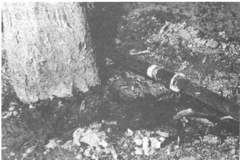
FIGURE 58 Trickle emitter dripping irrigation water. (F. K. Aljibury)
