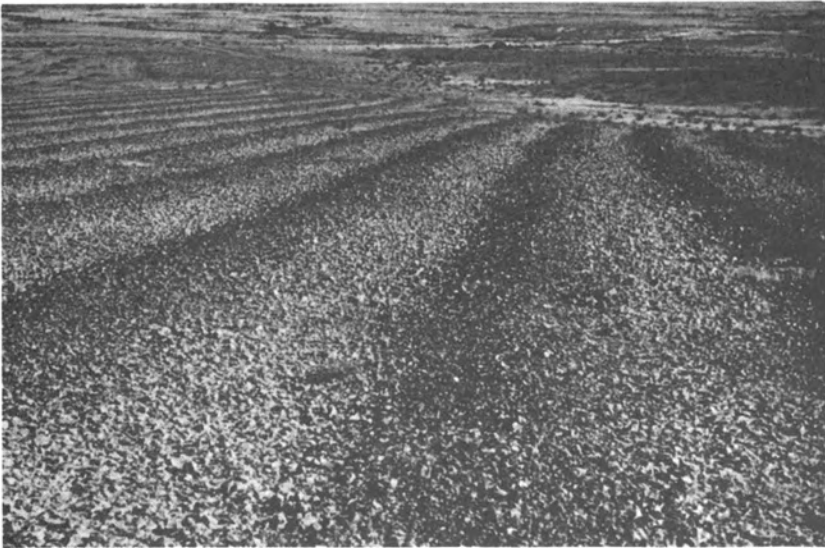
FIGURE 3 Ancient rainwater-harvesting system in the Negev. Gravel that covered the slopes has been moved aside, leaving a catchment that directs rainfall runoff to a farm in the valley. (M. Evenari)
