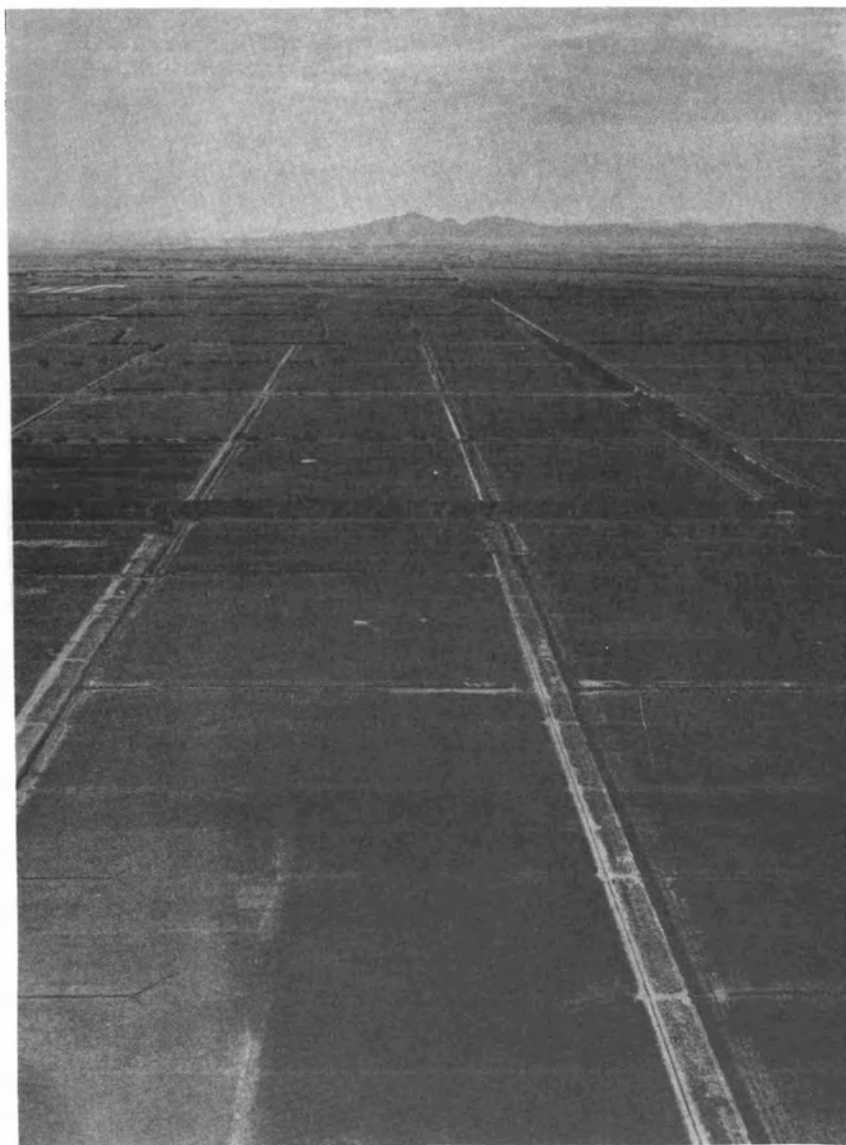
FIGURE 31 This Melbourne and Metropolitan Board of Works Sewerage Farm at Werribee, Australia, has long used treated sewage from the city of Melbourne as irrigation water. This formerly barren, arid, windswept plain is the major sewage-disposal facility, serving more than 1.5 million people. (Sewage flow averages 360 million l per day, 950 mld during rainy periods.) The farm grazes 15,000 cattle a year; 40,000-50,000 sheep are fattened during the spring and summer, resulting in the sale of 5,000 cattle, 36,000 sheep, and 250 bales of wool during an average year. (Melbourne and Metropolitan Board of Works)
