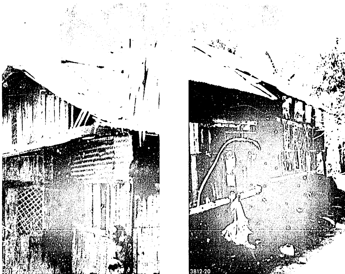
Figure 10. Typical Rural Housing in Bangladesh Showing Extensive Use of CGI Sheeting for Roofing and Walls. Note land eroded away due to flooding.
