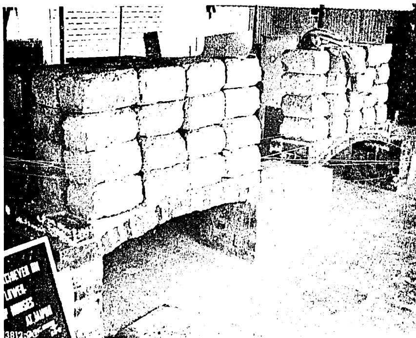
Figure 12. Illustration of Flat-Arch Roof System of the Central Building and Research Institute, Roorkee, India. Materials are brick and gypsum.
