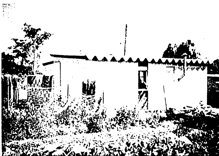
Figure 14. Cement-Asbestos Roofing Manufactured by the TAP Company On the Outskirts of Lusaka, Zambia. Shown on the Loading Dock at the Factory and Installed on a Low-Cost House.
