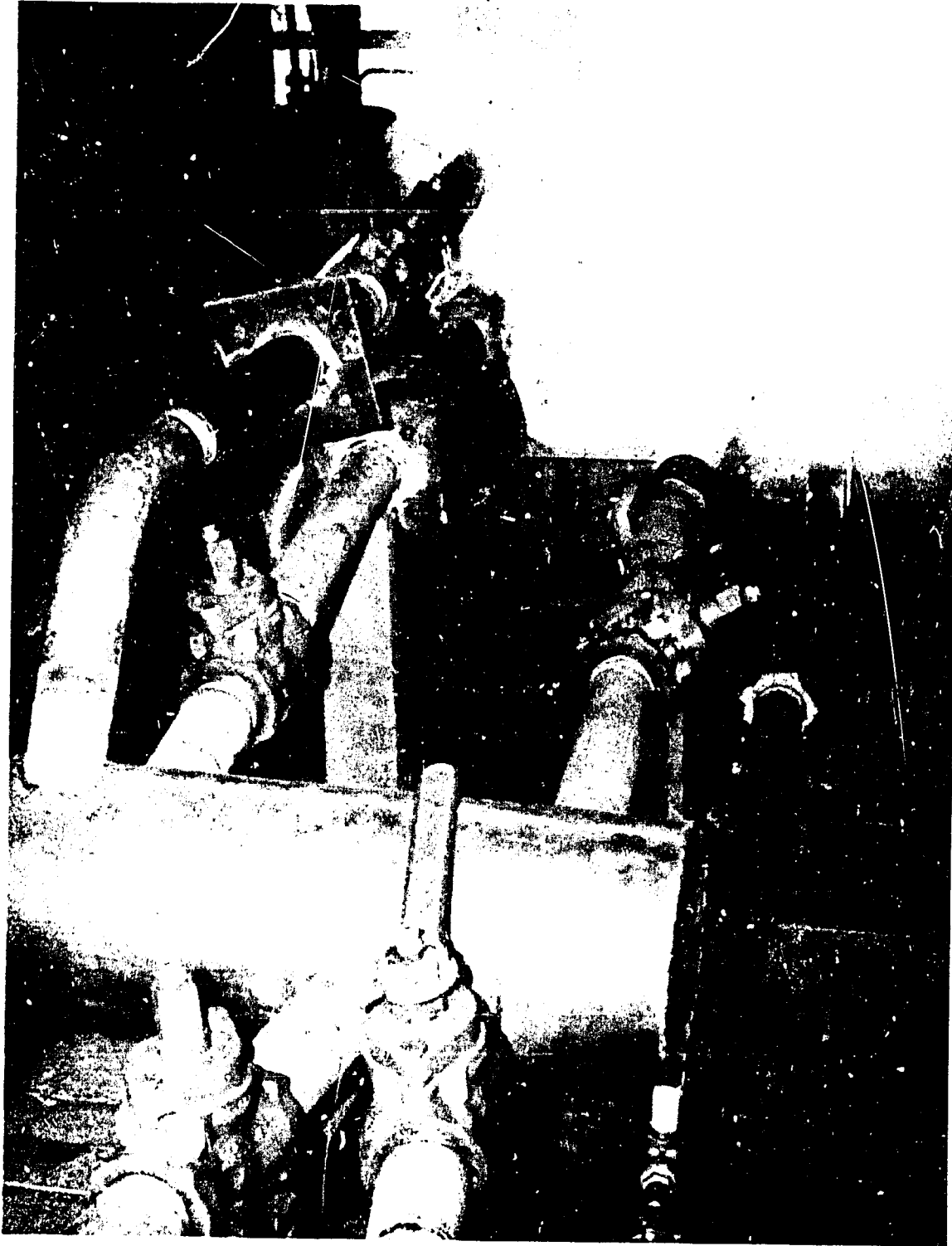
View of Manifold, Scavanger Fans and Top of the Reactors (background), while System is in operation.
