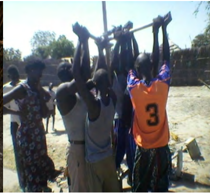
Pump minders on repairing a hand pump
