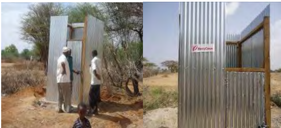
Some of the toilets constructed in Wajir Bor community through cash-for-work
