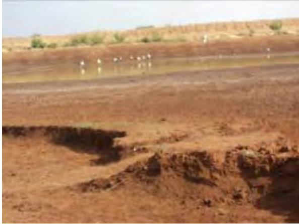
a) Dam de-silting and deepening at Tulatula
