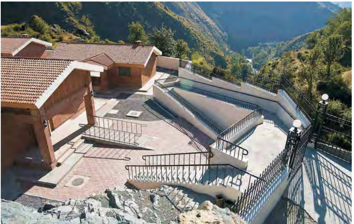
Basic Health Unit Kala Mula. As with most of the buildings in the project, they are accessible to the disabled as the ramp here indicates.
