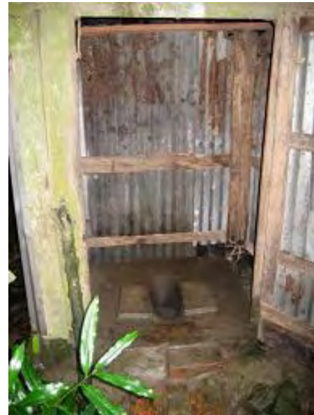
Figure 8: Toilet with a broken water seal, middle class house
