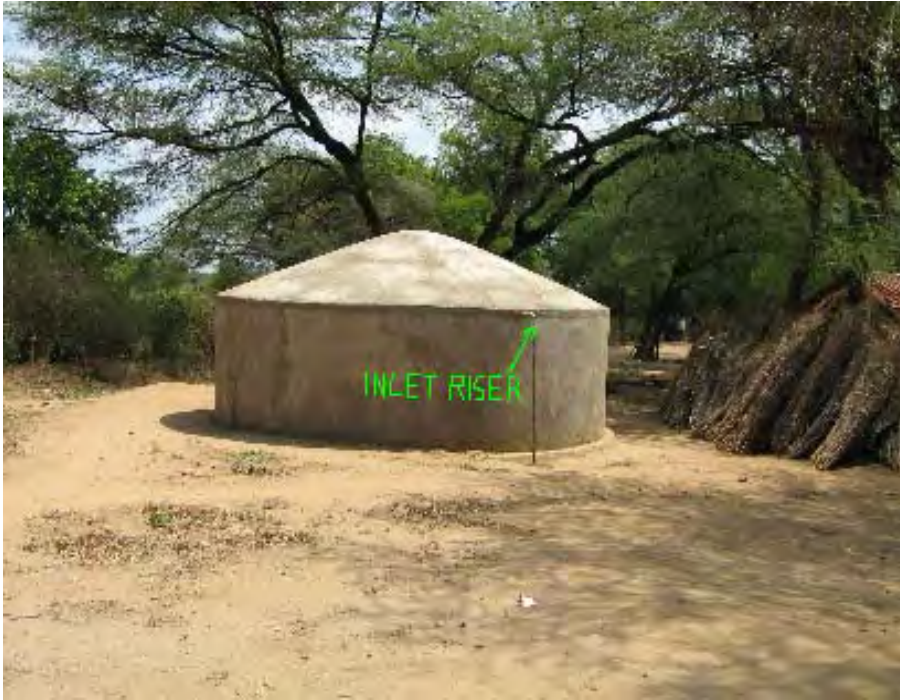
One of the two ferro-cement storage tanks in Kimatong.
