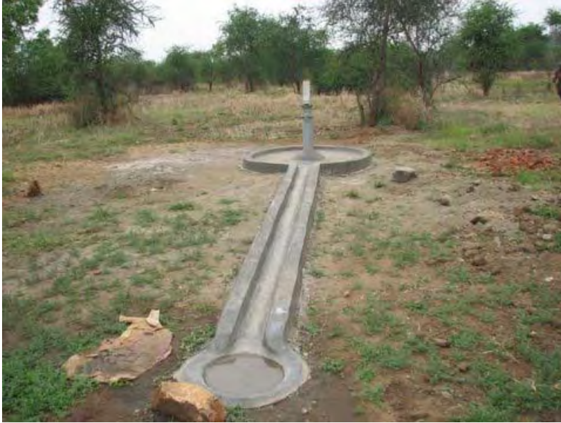
A newly constructed borehole in Lafon.
