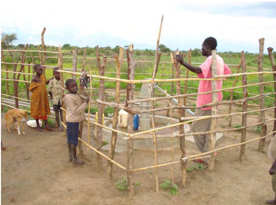
New borehole in Ikotos County.
