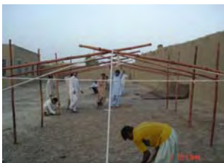
Team constructing shelter house
