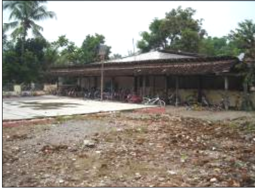
SDN 01 Somopuro, Klaten, before the reconstruction process, June 2008
