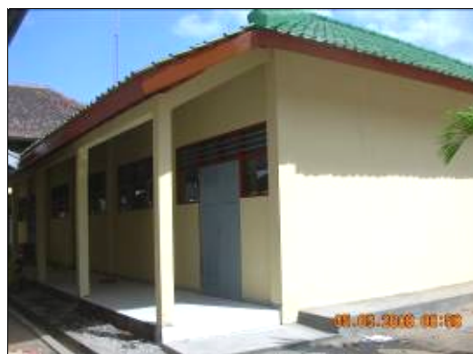
SMPN 15 Yogyakarta, after the reconstruction process, September 2008
