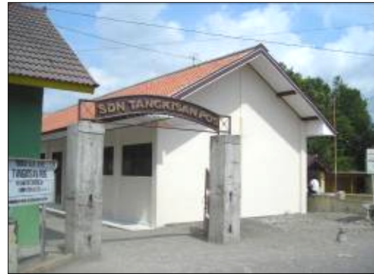
SDN Tangkisan Pos, Klaten, after the reconstruction process, September 2008
