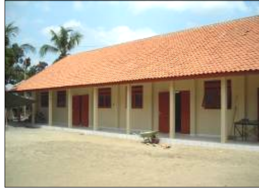
SDN 01 Somopuro, Klaten, after the reconstruction process, September 2008
