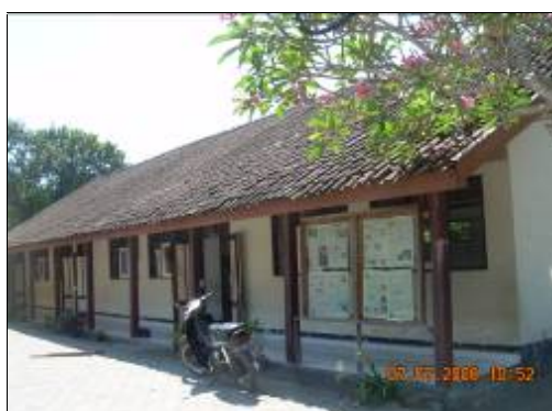
SDN Salakan Lor, Sleman, before the rehabilitation process, July 2008
