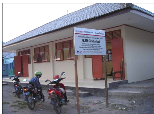
PKBM Gita Lestari, Sleman, after the reconstruction process, September 2008
