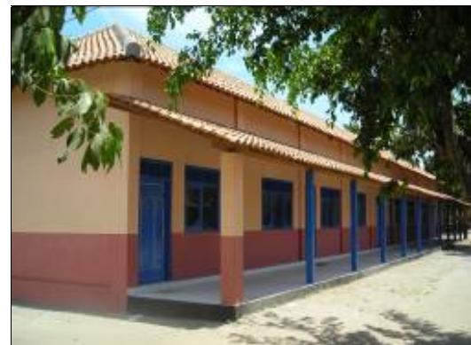
SDN 01 Granting, Klaten, after the rehabilitation process, September 2008
