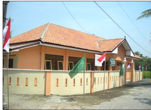
MTs Al Falaah, Bantul, after the rehabilitation process, August 2008
