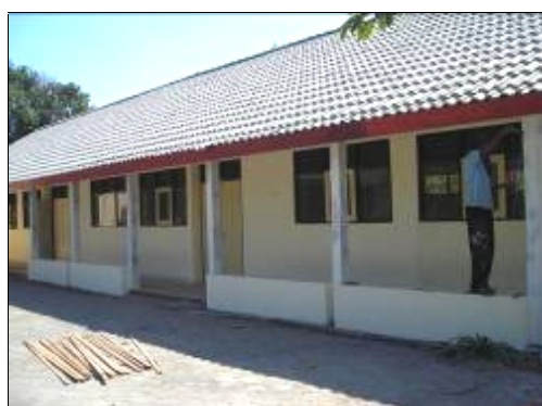
SDN Salakan Lor, Sleman, after the rehabilitation process, September 2008
