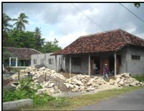
MTs Al Falaah, before the rehabilitation process, May 2008
