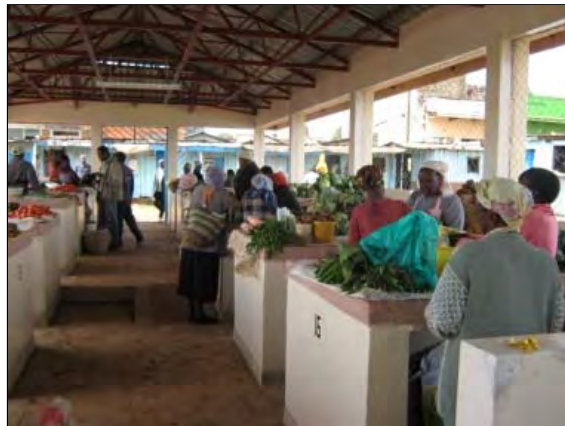
The renovated Burnt Forest Market is again open for business.
