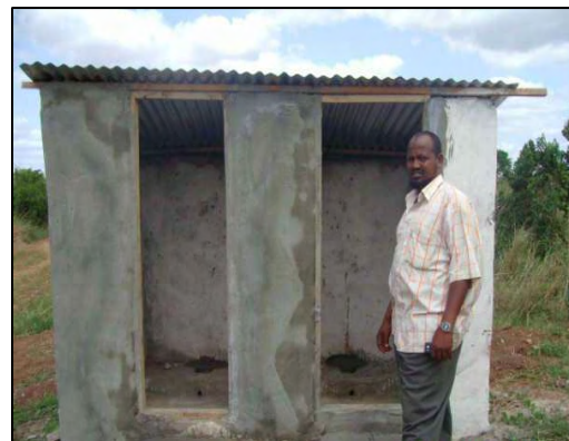
Constructing the pit latrines
