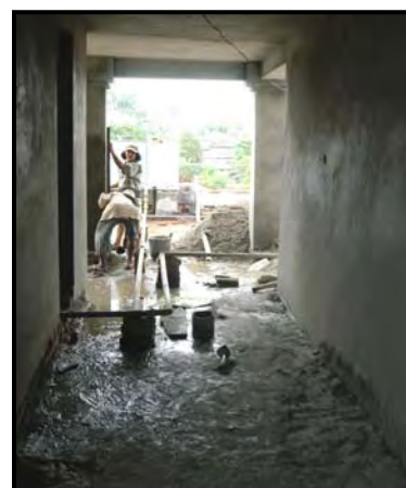
Repairs and Maintenance at Patan Appellate Court
