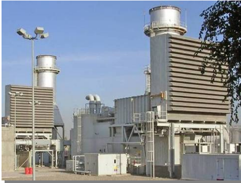
Newly constructed Baghdad South: Units 1A and 1B
