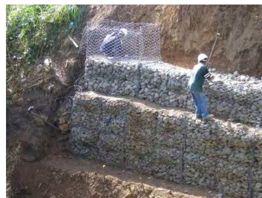
Above: Big Hole #2 Gabion Basket Retaining Wall construction.
