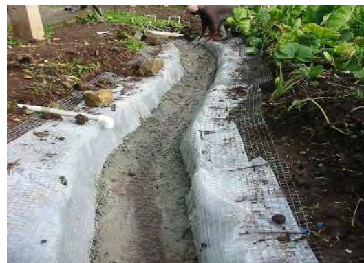
Above: The “STAR drains” system developed by MoSSaiC provides low-cost temporary drainage from house gutters and waste pipes to main drains. This intervention reduces water inputs into surrounding soil which can saturate soils and increase landslide risks.
