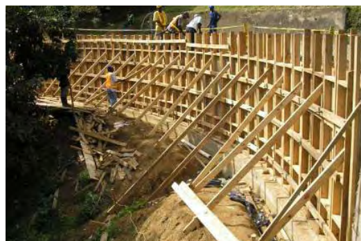
Above: Good Wood Concrete Retaining construction.
