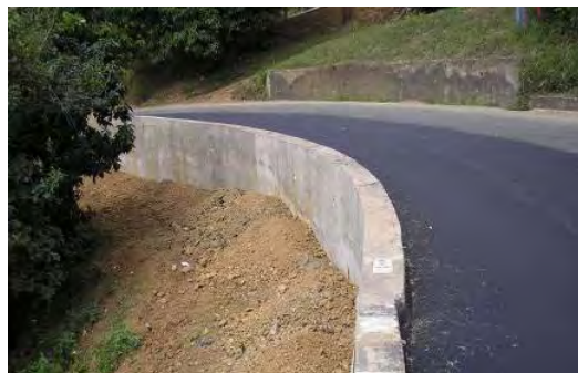
Above: Good Wood Concrete Retaining wall complete.
