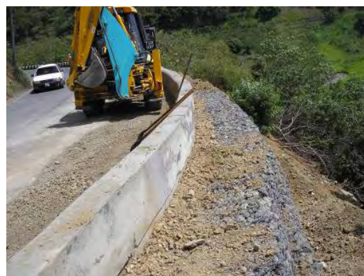
Above: Big Hole #1 Gabion Basket Retaining Wall complete.
