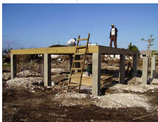
Above & Below: PADCO constructed the houses on stilts to mitigate against future storm surge in this low lying community.
