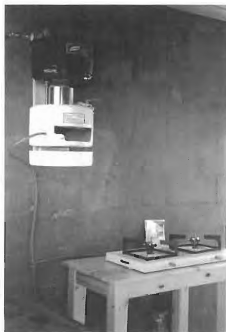
Amazing Amanzi water heating system
