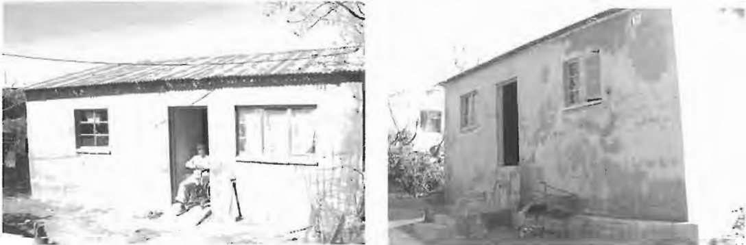
External plaster and weather stripping of joinery and installation of a ceiling
