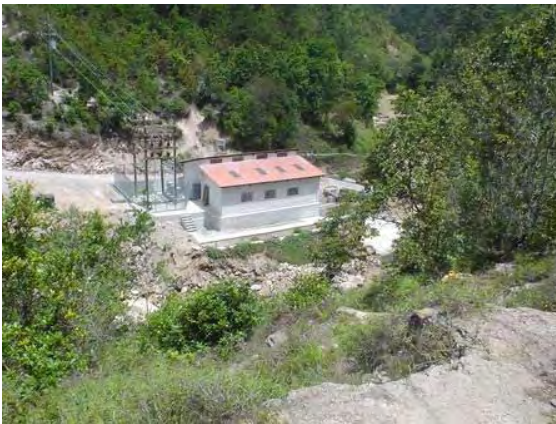
E+Co funded, 485 kW La Esperanza Hydroelectric project, Honduras
