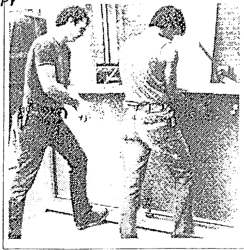
2 Remove the braces from around the hardware while holding the door so that it does not fall open. CAUTION: Door is not locked during shipment
