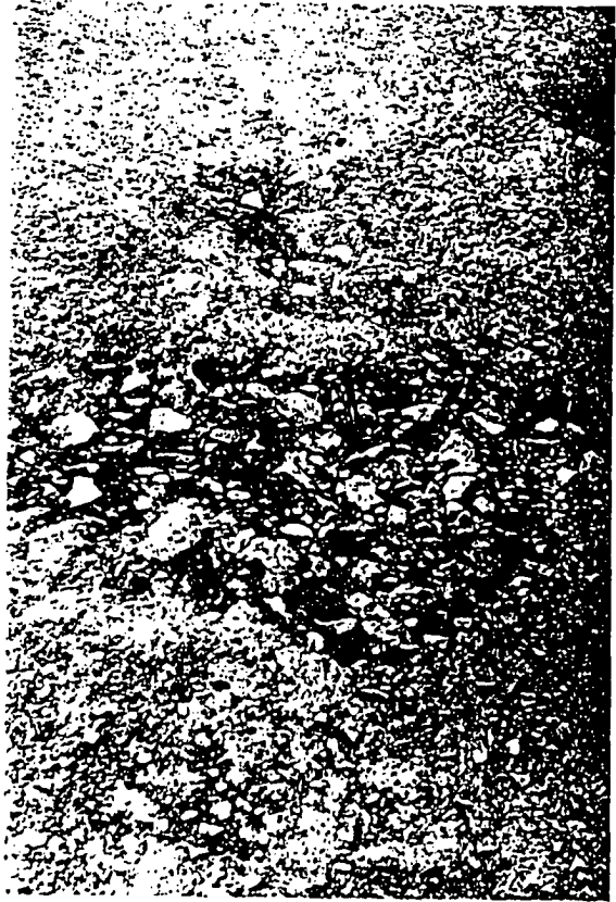
POTHOLES DEVELOPING DUE TO SEWERAGE WATER (CLOSE VIEW)
