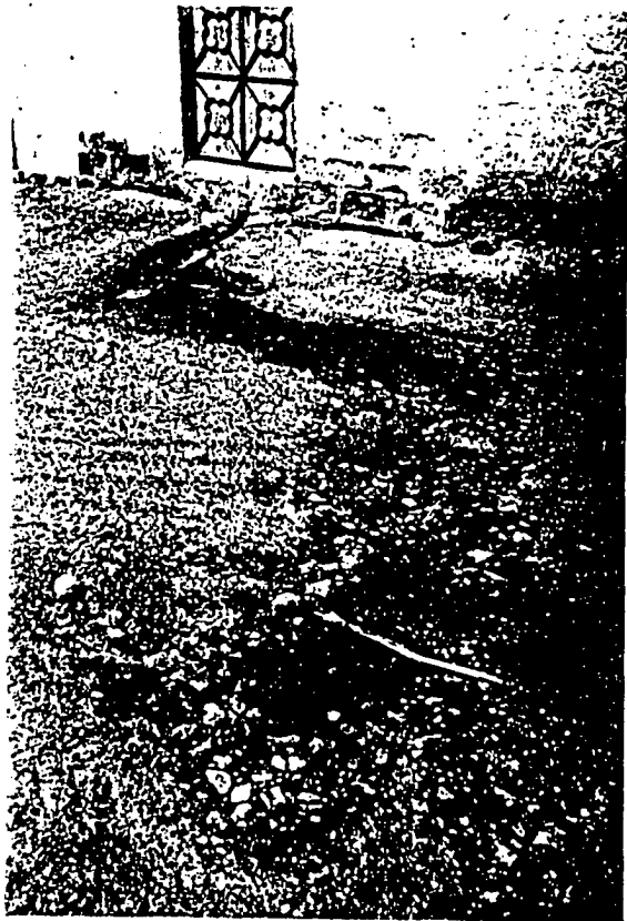
SEWERAGE WATER COMING ON SURFACE OF THE ROAD DUE TO NON-EXISTENCE OF DRAINAGE
