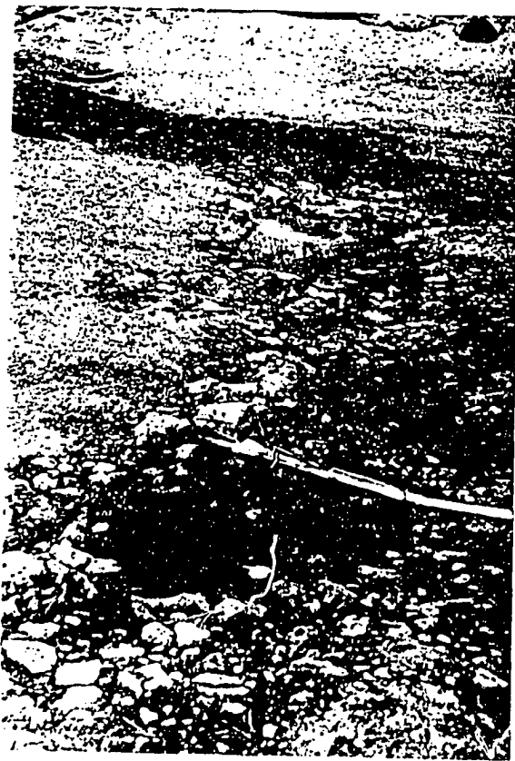
POTHOLE DEVELOPED DUE TO SEWERAGE WATER
