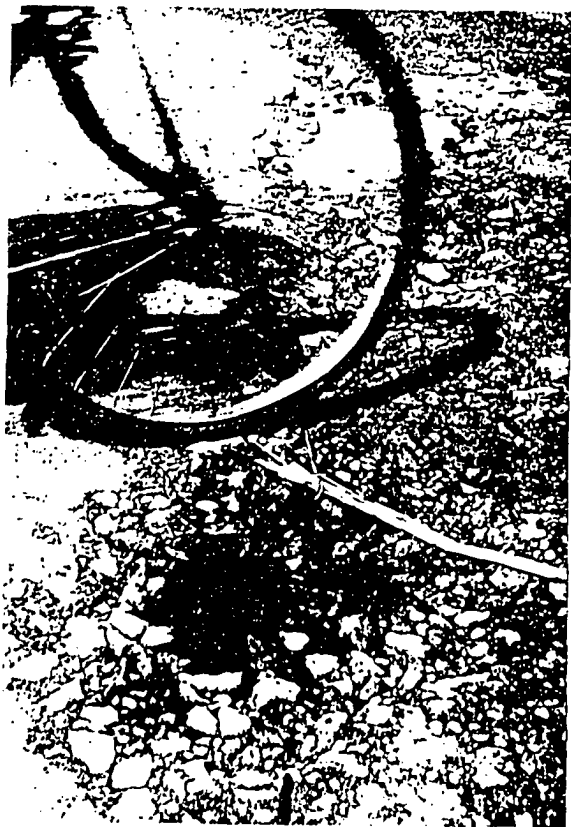
SEWERAGE WATER COMING ON SURFACE OF THE ROAD DUE TO NON-EXISTENCE OF DRAINAGE
