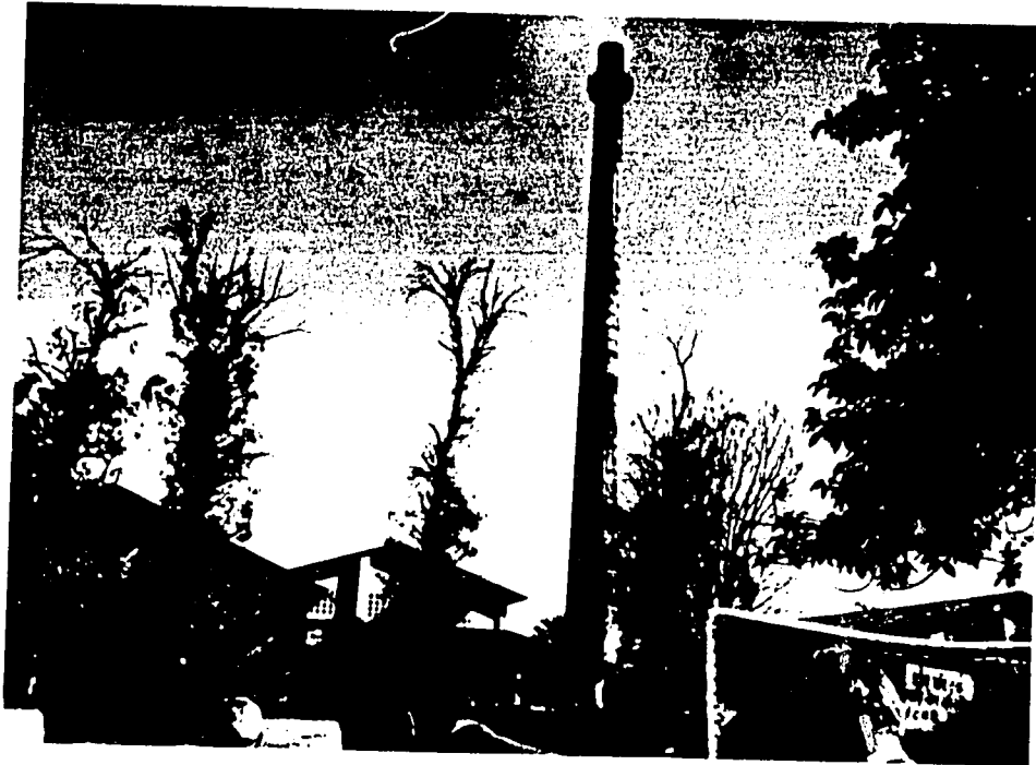
7. Smoke Stack of Hirisiddhi Brick Factory in Kathmandu
