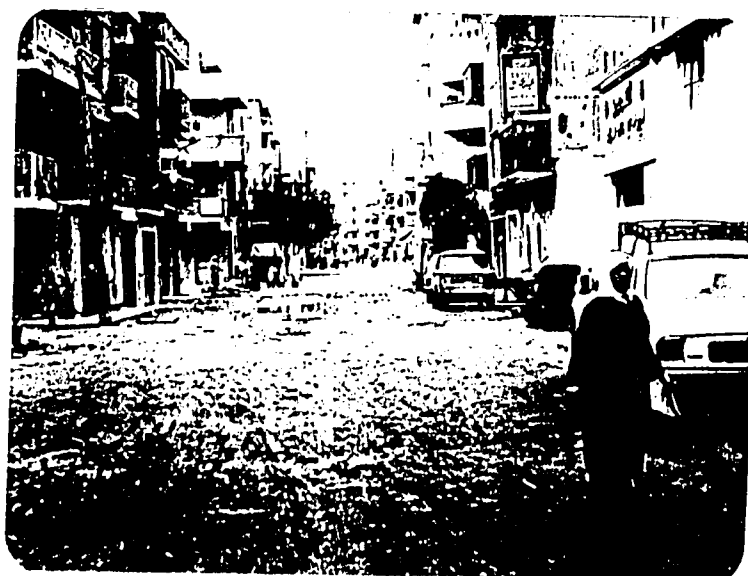
Bad-paved Streets in Giza City Figure 5
