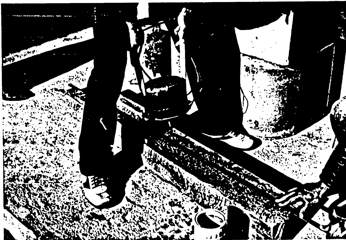
PROJECT REGIONAL COMPLEX - IMPROVISED ELECTRIC DRILL BEING USED IN THE LATRINE FACTORY.
