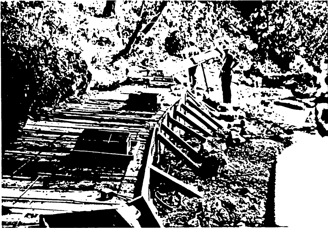
SPRING CAPPING PROJECT CALLED JUTACAJ UNDER CONSTRUCTION. IT WILL SERVE THE COMMUNITIES OF JUTACAJ, RACANA, SICALBE AND JOSE SIGUILA IN THE DEPARTMENT OF TOTONICAPAN. THERE WILL BE 220 HOUSEHOLD CONNECTIONS. THE LENGTH OF THE DISTRIBUTION LINE WILL BE 35 KILOMETERS. IT WILL SERVE 1,400 PEOPLE.
