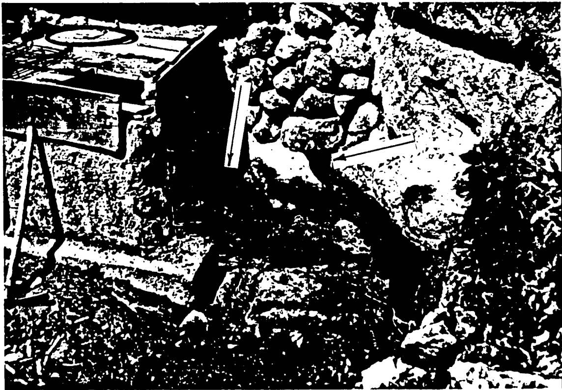
THIS PICTURE SHOWS THE END OF THE COLLECTION BOX. THE TWO ARROWS INDICATE THE TWO MAIN SPRING VEINS WHICH WILL BE FEEDING THE WATER DISTRIBUTION TANK.
