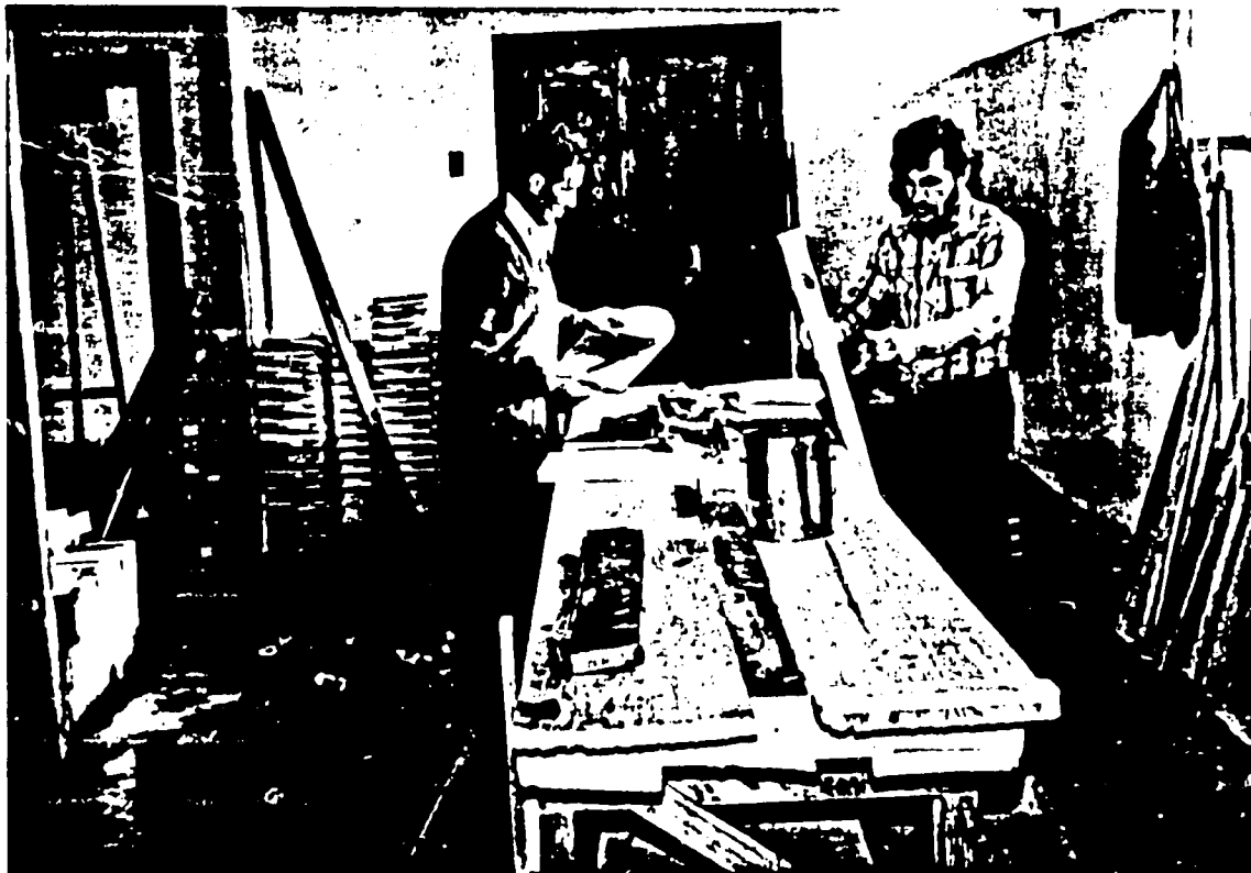
PROJECT REGIONAL COMPLEX - CARPENTRY SHOP MANUFACTURING LATRINE SEAT TOPS.
